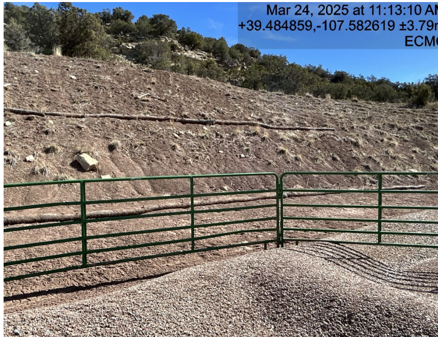
Waddles failing/ cut slope erosion
