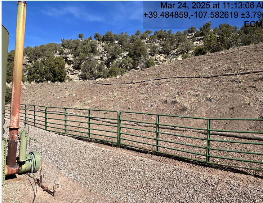
Waddles failing/ cut slope erosion
