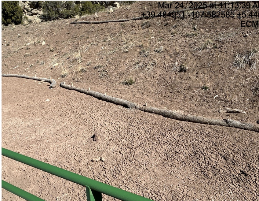
Waddles failing/ cut slope erosion
