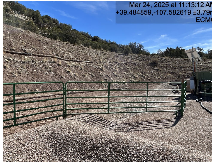
Waddles failing/ cut slope erosion
