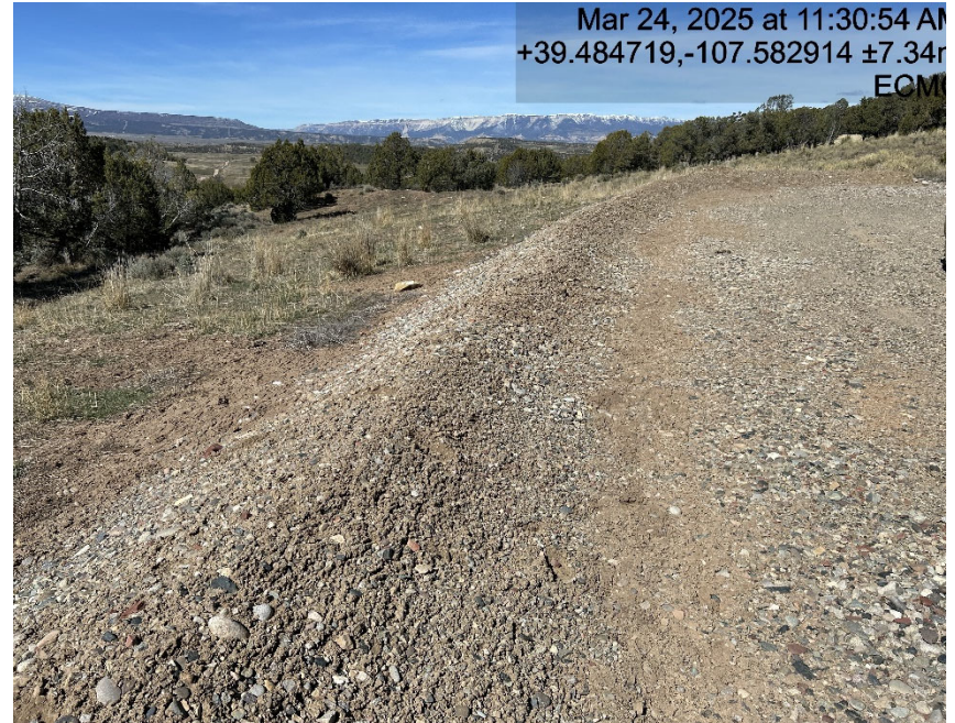
Berm is not compacted
