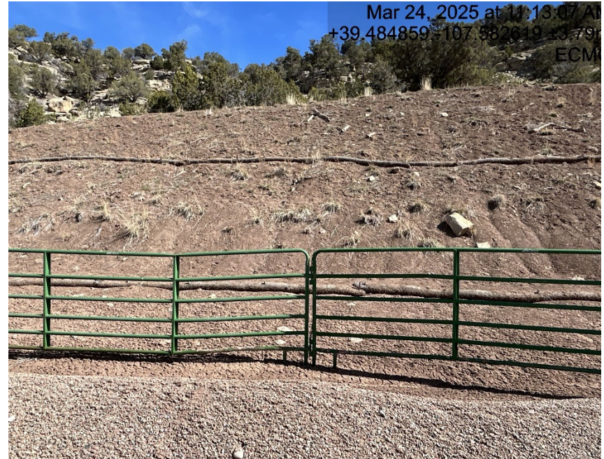
Waddles failing/ cut slope erosion
