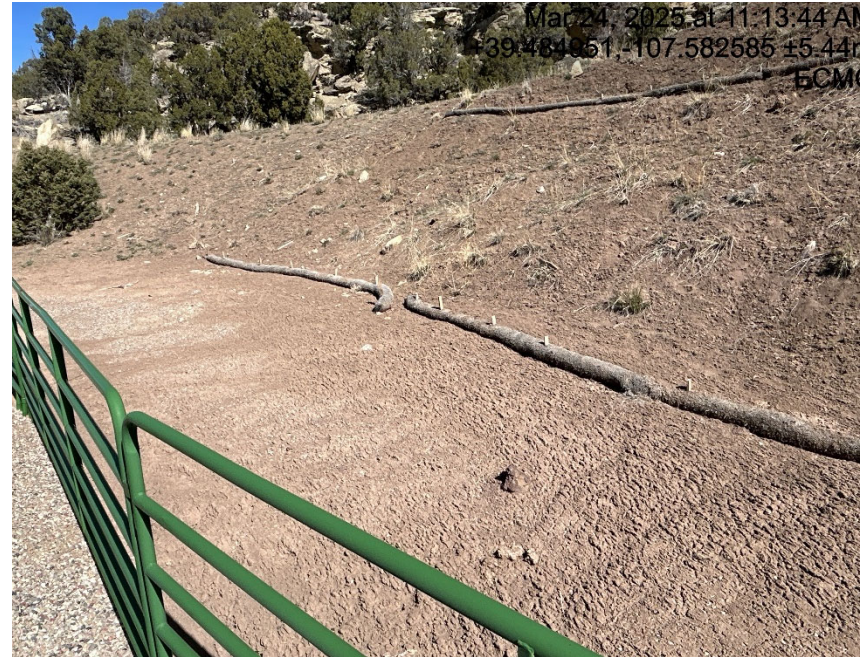
Waddles failing/ cut slope erosion
