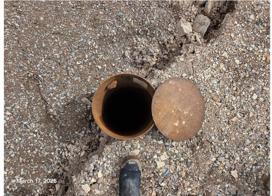
**Photo 3:** Photos examples showing a rat, mouse, or other bore hole that has not been properly closed/backfilled pursuant to 1003 requirements.
