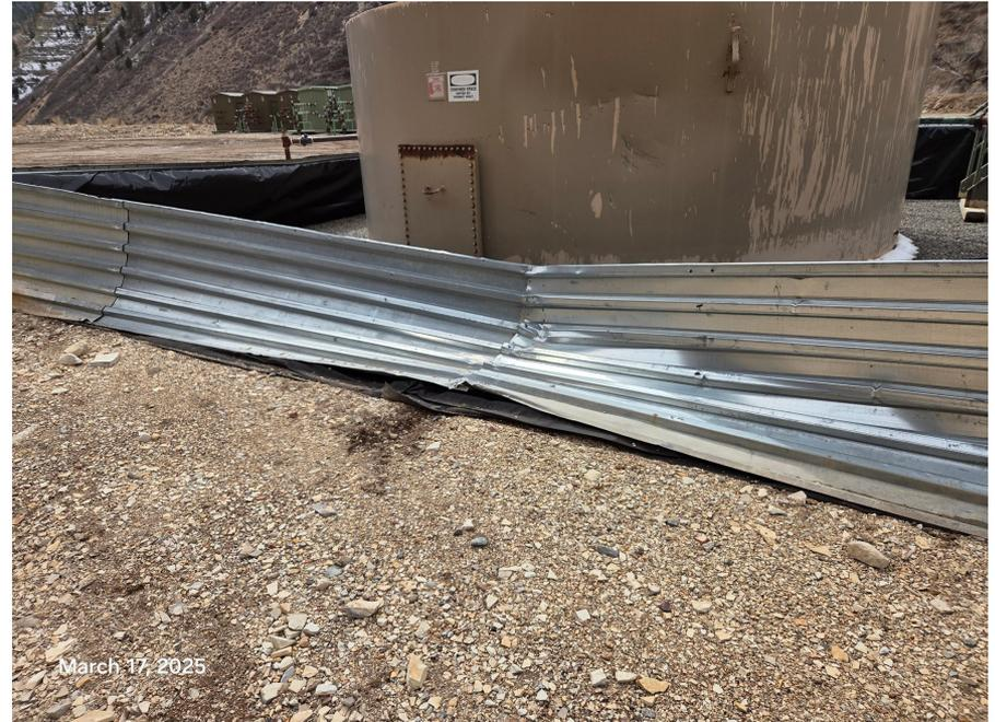
**Photo 5:** Photo taken from the tank facility on the east end of the Location. Photo shows containment BMP has received significant damage, and it is not clear if BMP is in proper functioning condition, or sufficiently impervious to contain a spill or release.
