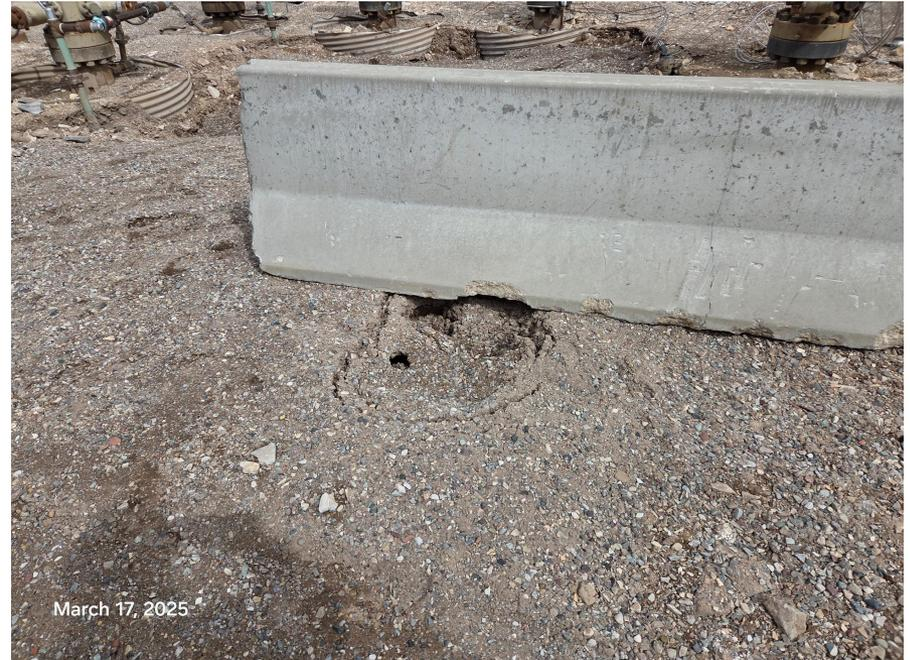
**Photo 1:** Photos examples showing subsidence issues observed at the wells on Location.
