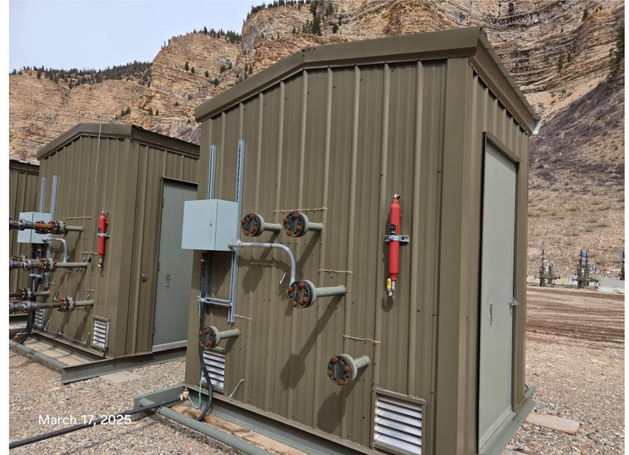
**Photo 6:** Photo taken from the southwest end of the Location. Photo shows unused Gas Meter/Lift and riser equipment; equipment requires removal pursuant to Rule 606
