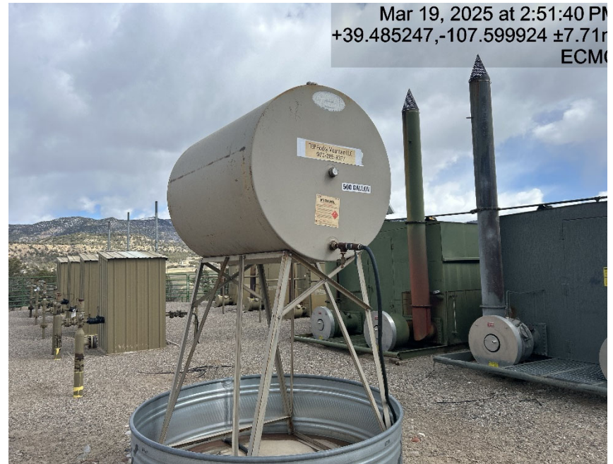
Methanol tank in containment
