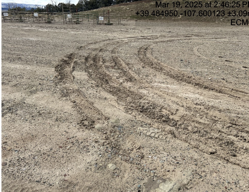
Location shows sins of lack of stabilization/ compaction
