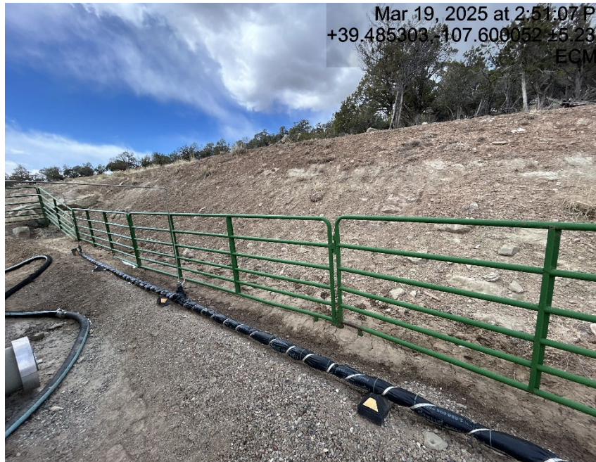
Cut slope not stabilized and show areas of erosion.
