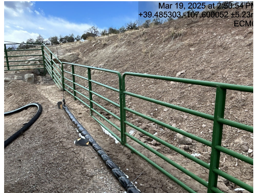
Cut slope not stabilized and show areas of erosion.
