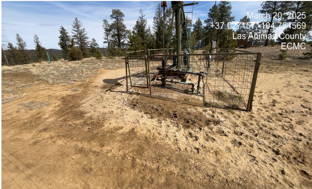
Photo 4. There is wet stained soil at the wellhead from a PW leak that needs to be cleaned up. Ensure leak is controlled.
