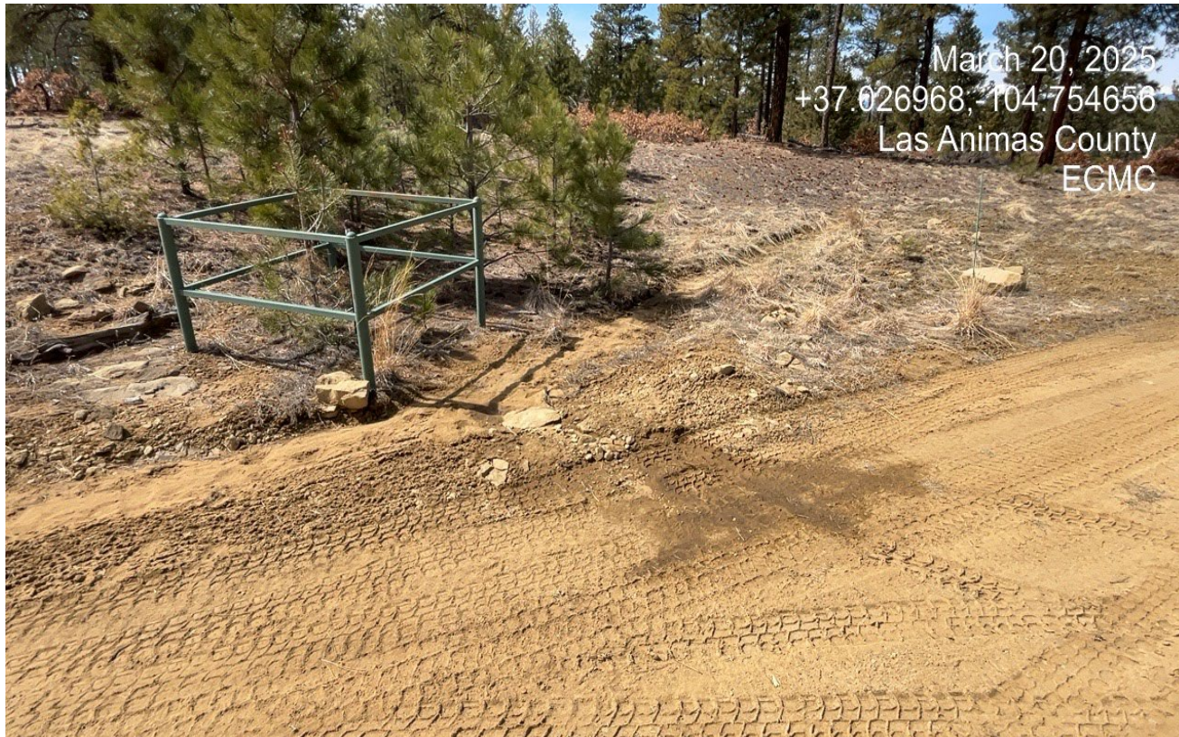
Photo 2. There is stained soil at this flowline valve that needs to be cleaned up.
