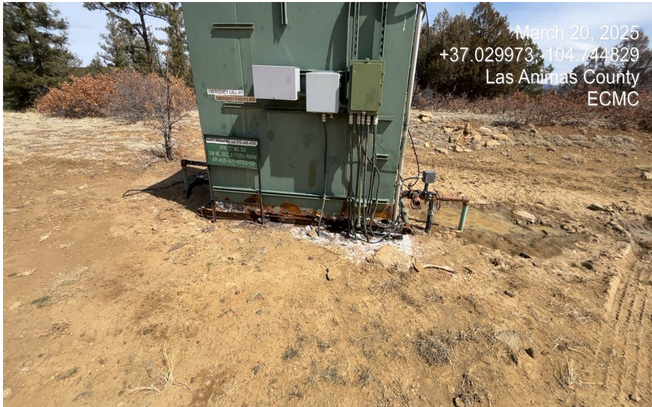
Photo 3. There is a dripping water leak at the meter shed. The base of the meter shed is all rusted out from the ongoing leak.
