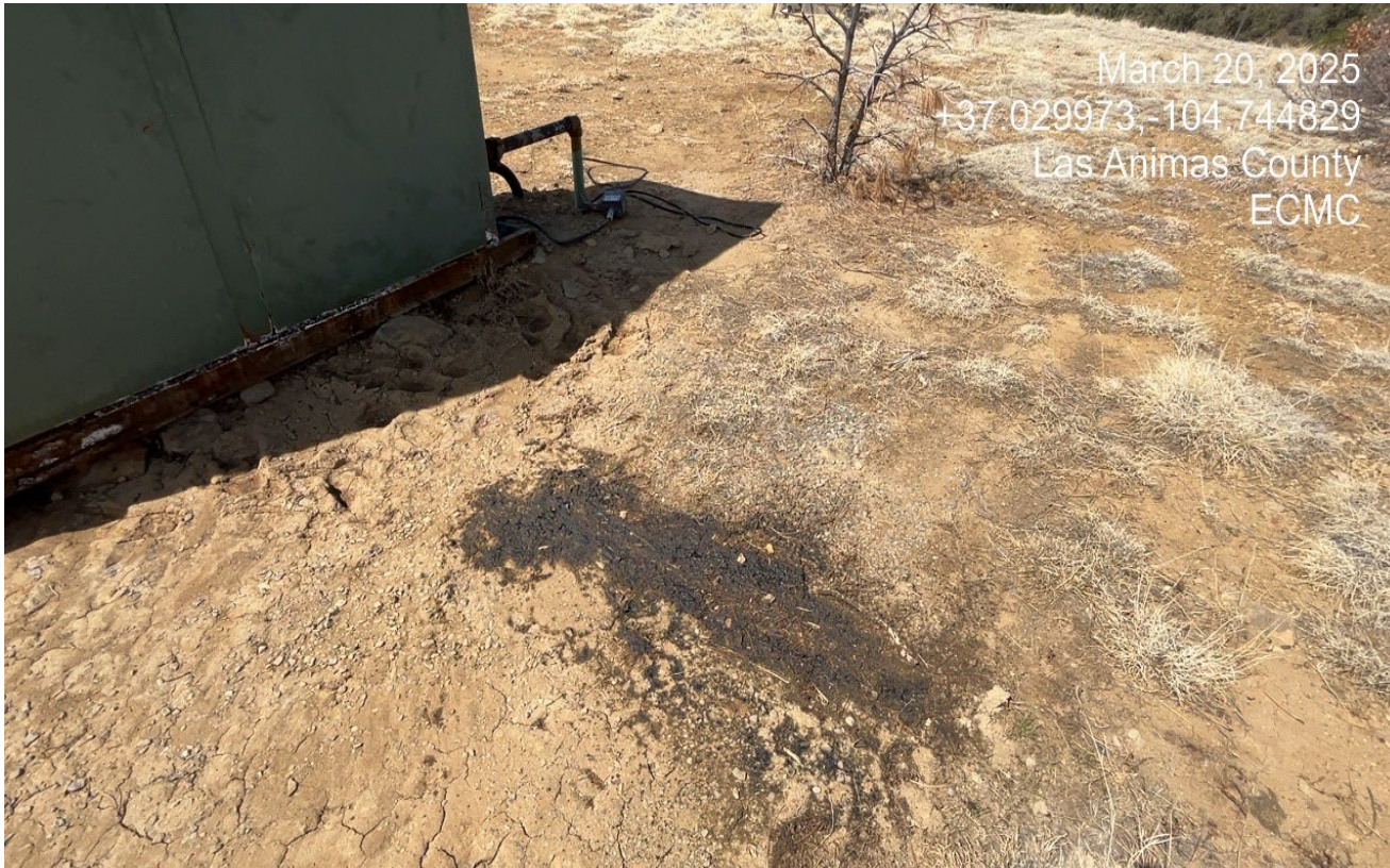
Photo 4. There is a hydrocarbon stain at the backside of the meter shed that needs to be cleaned up..
