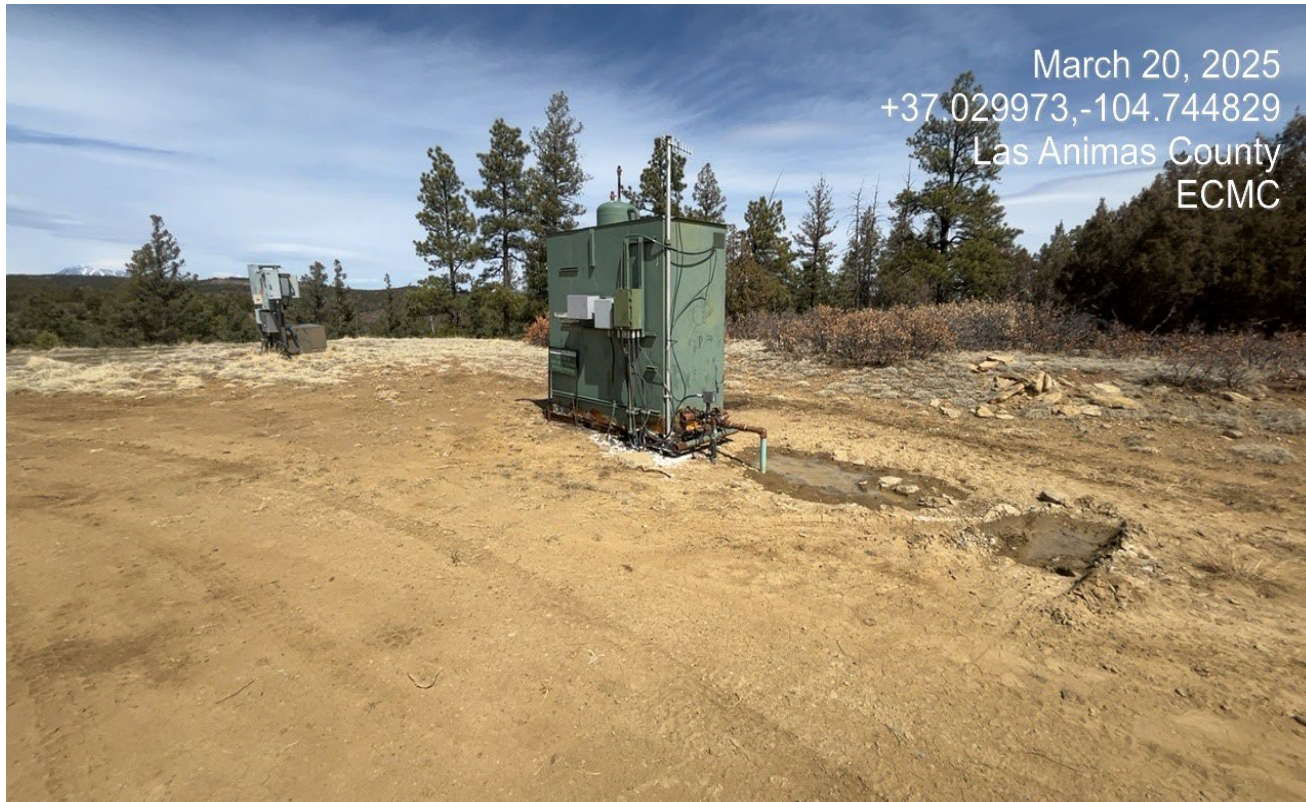
Photo 2. Facing northeast toward the meter shed. There is a produced water leak coming from the meter shed that needs to be fixed and cleaned up.
