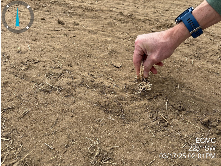
Photo 11. Photo taken from the western portion of the access road. Photo illustrates the Operator has only grubbed the access road and has not salvaged topsoil.
