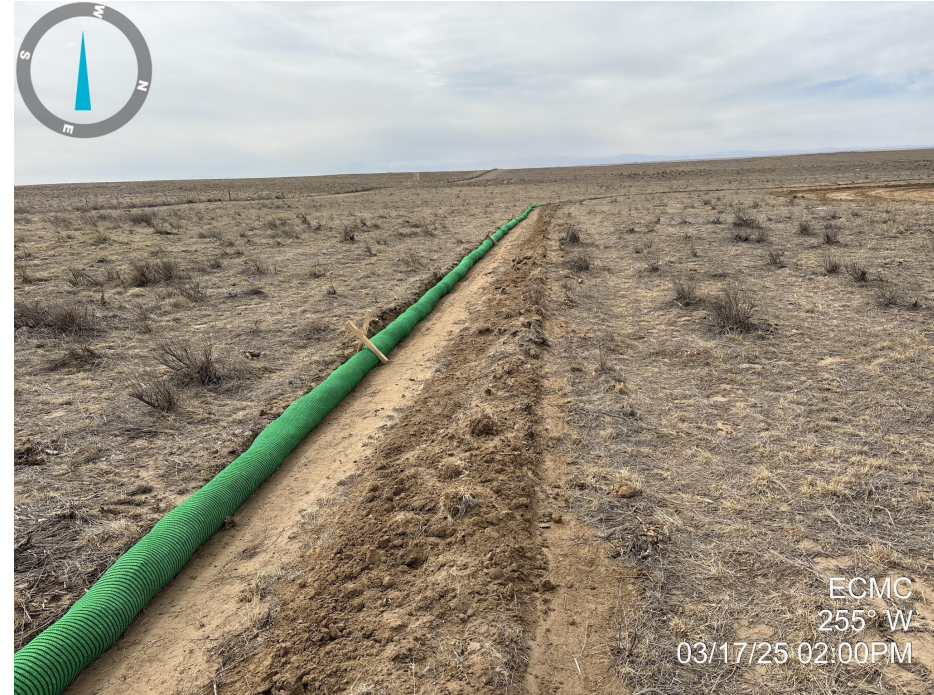
Photo 2. Photo taken from the southern perimeter of the site, facing West. Photo illustrates that a temporary BMP has been installed along the perimeter of the site.
