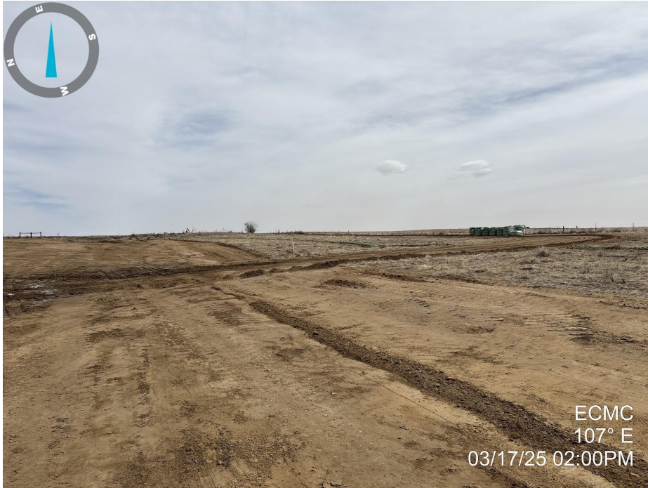
Photo 1. Photo taken from the southern perimeter of the site, near the location's entrance from the access road, facing East. Photo illustrates that the Operator has installed a ditch BMP.
