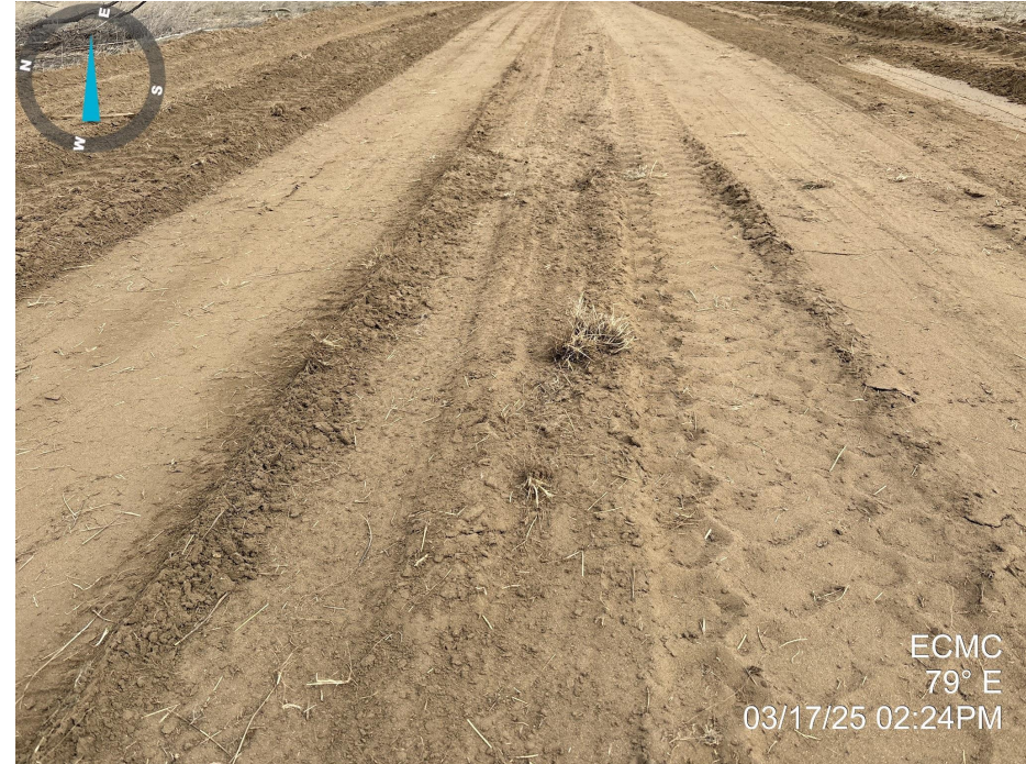
Photo 10. Photo taken from the previous photo location, along the access road, facing East. The photo illustrates vegetation and topsoil being used as fill material to construct the access road.
