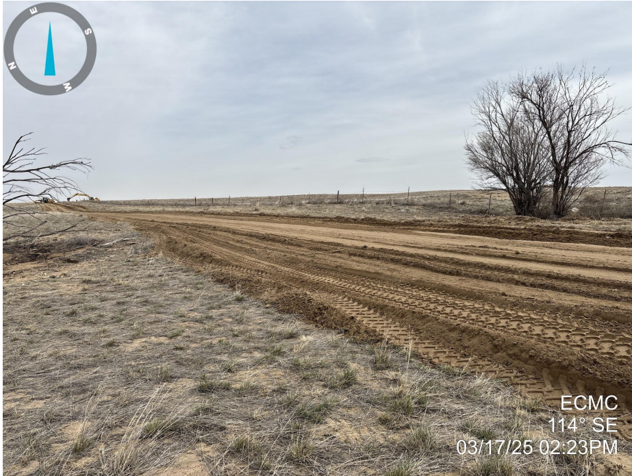
Photo 9. Photo taken along a portion of the western access road. Photo illustrates Operator is using access road topsoil as fill material and there are no access road BMPs.
