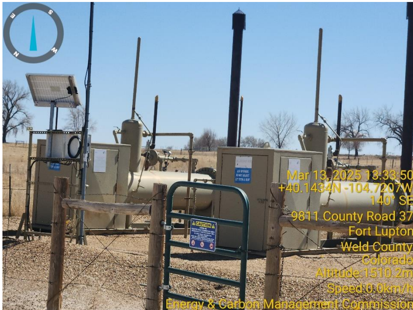
Photo 7 Horizontal heated Separators
