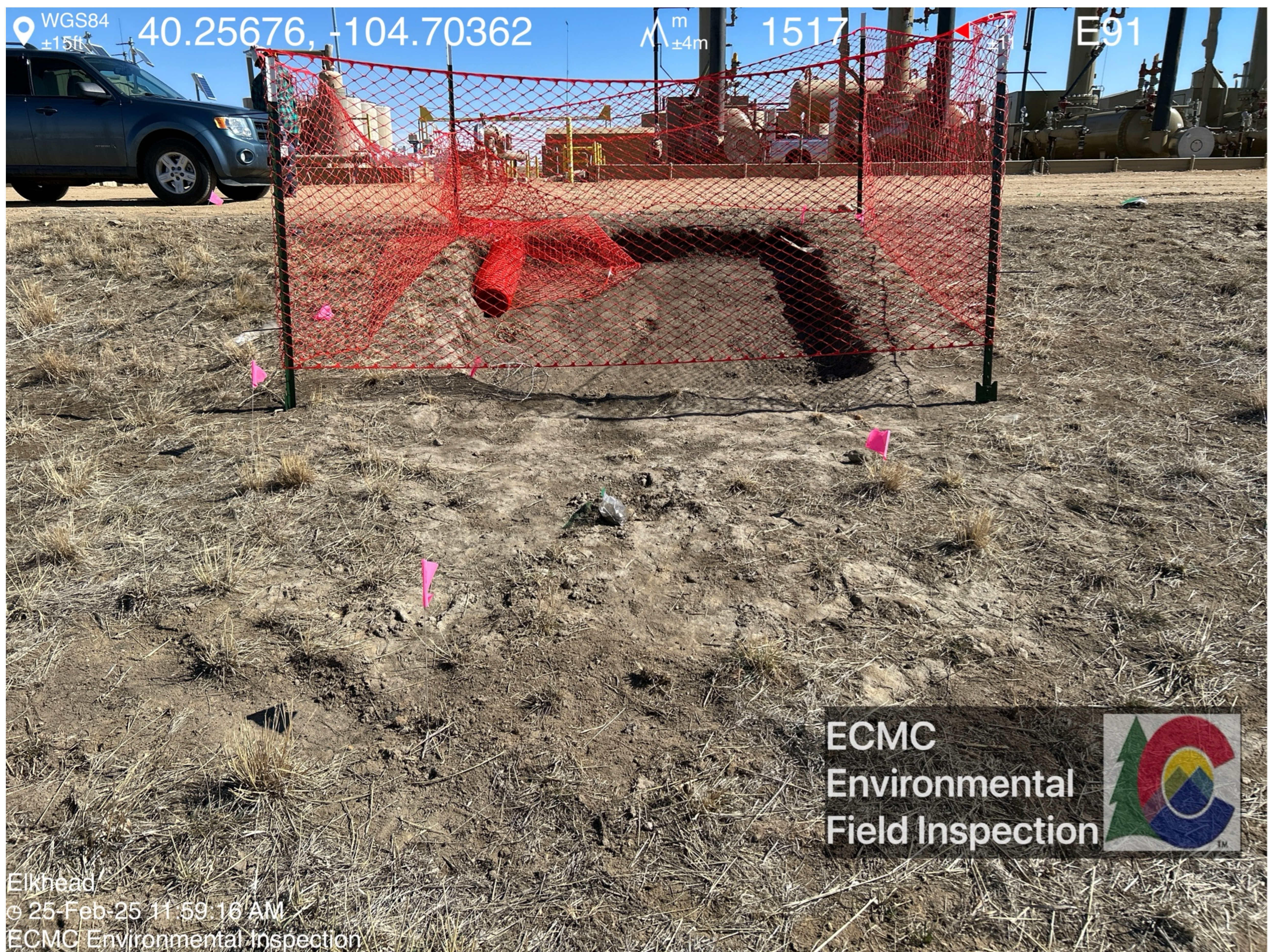
Pink flags are visible in an area of impacted vegetation and soil at the spill location. Multiple plastic bags containing soil are visible.
