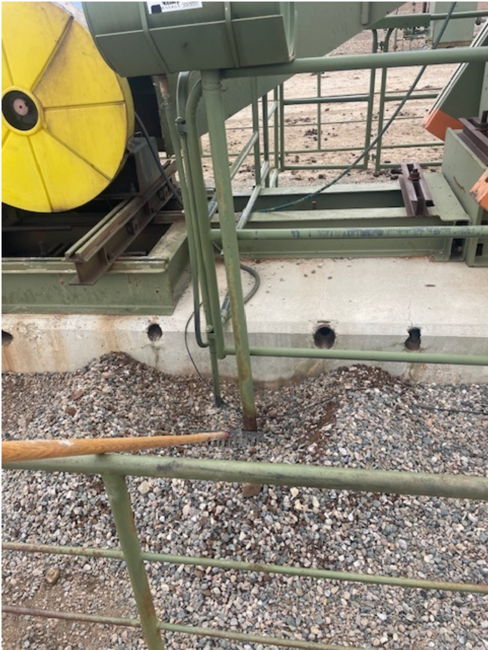
Containment was built around oil day tank.
