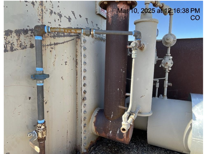
Photo # 1724 PRV vent line does not comply with CECMC rules
