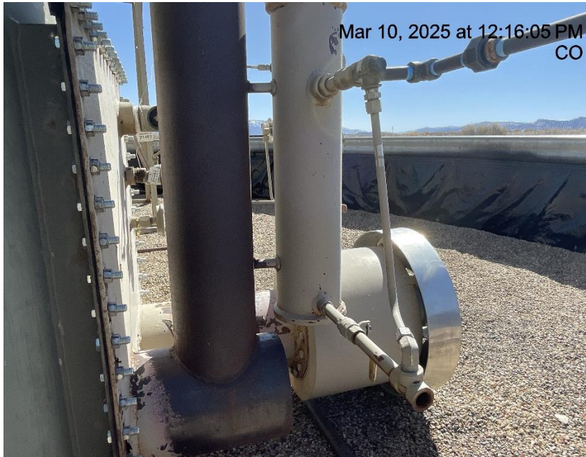
Photo # 1723 PRV vent line does not comply with CECMC rules
