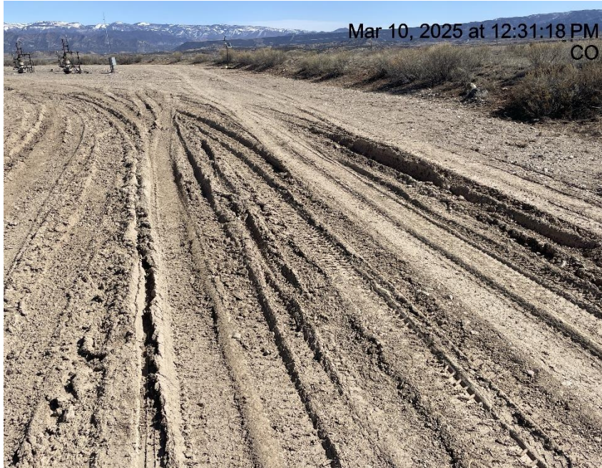
Photo # 1725 Lack of stabilization/compaction
