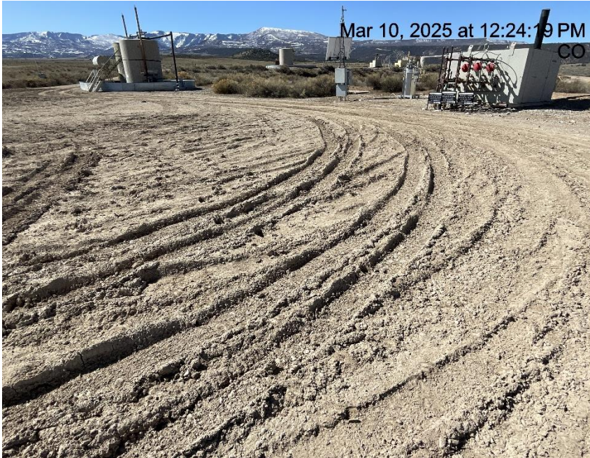
Photo # 1731 Lack of stabilization/compaction
