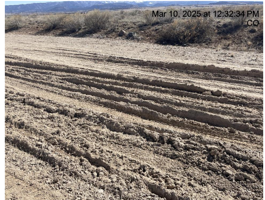
Photo # 1728 Lack of stabilization/compaction
