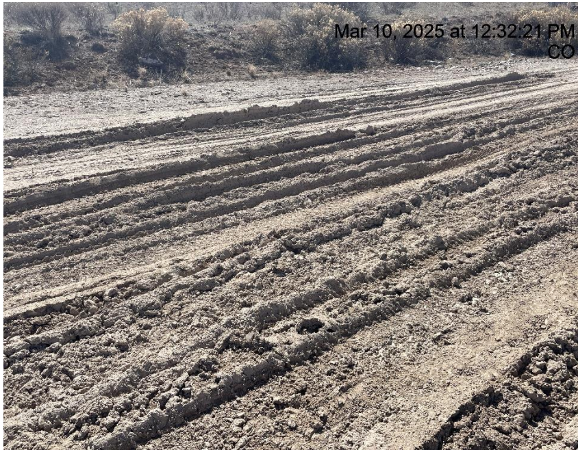
Photo # 1727 Lack of stabilization/compaction
