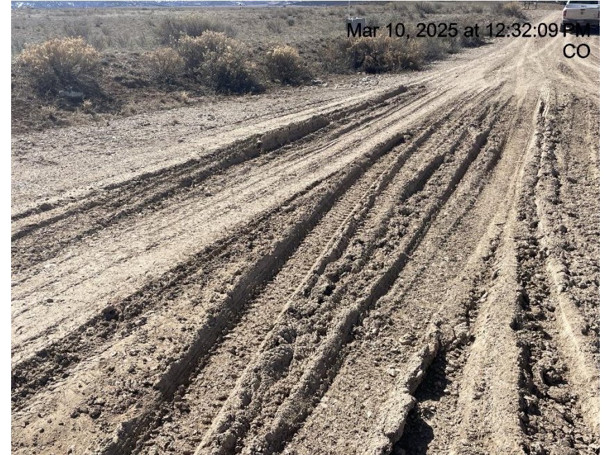
Photo # 1726 Lack of stabilization/compaction
