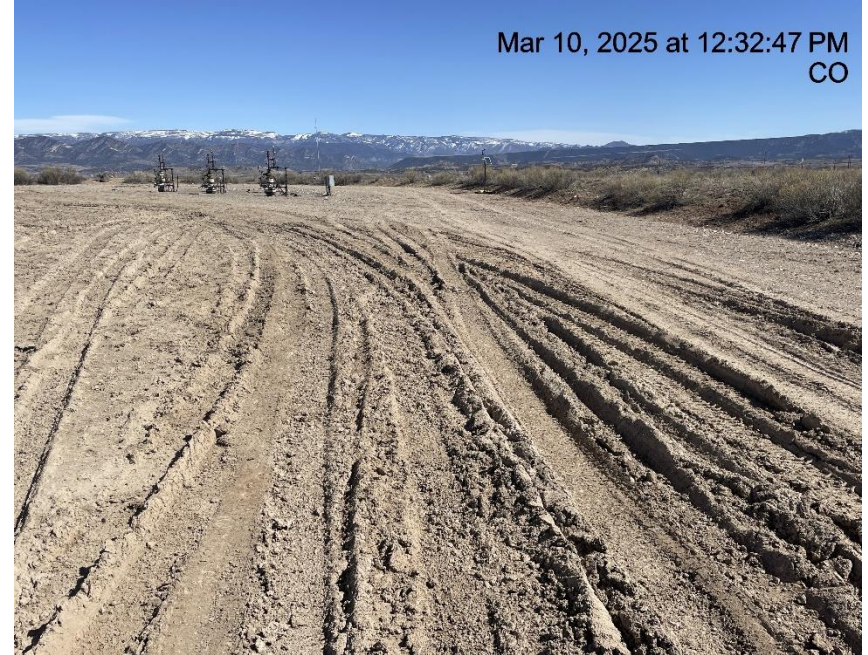
Photo # 1730 Lack of stabilization/compaction
