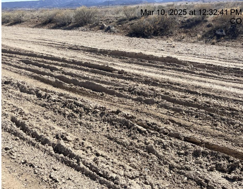
Photo # 1729 Lack of stabilization/compaction
