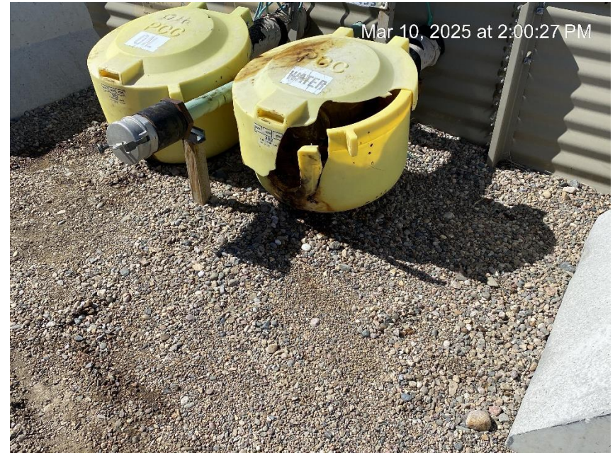
Damaged loadout pot
