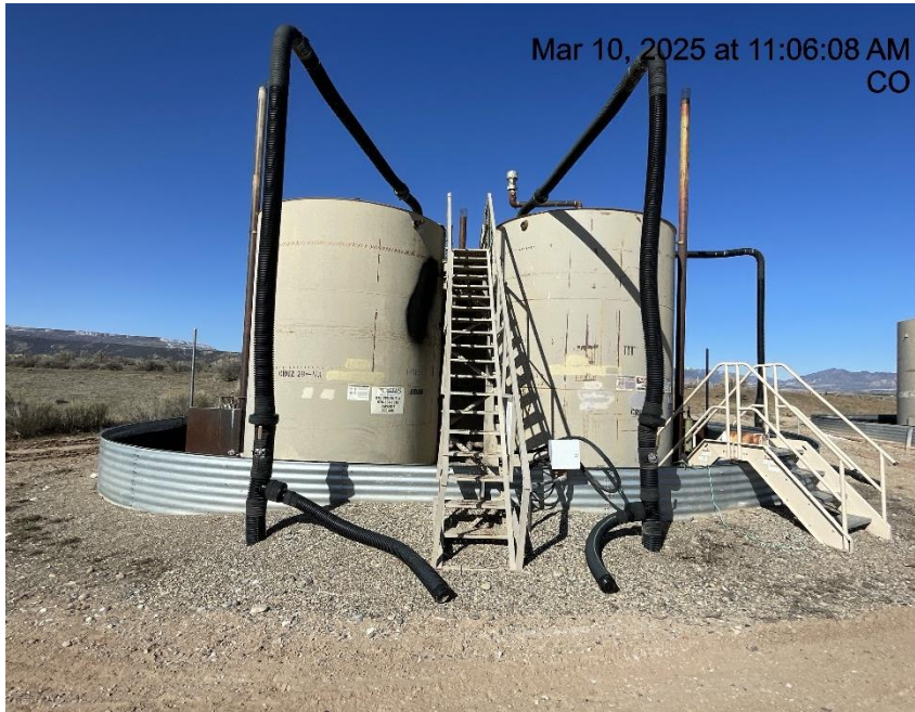
Photo # 1567 Battery lacks required signage/not in compliance with CECMC rules
