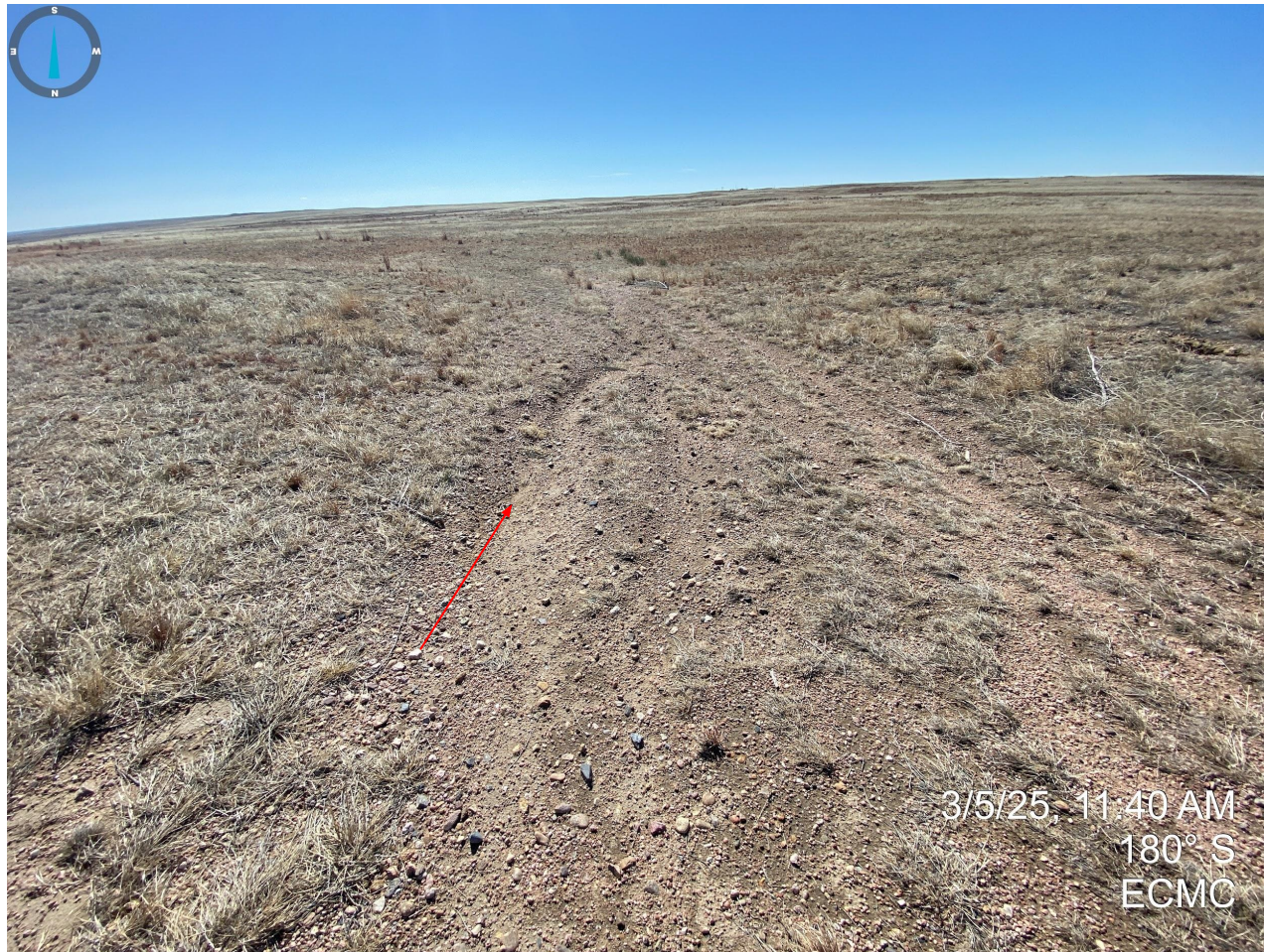
Photo 1. Stormwater erosion degradation observed at the former location entrance/access road, which does not appear to have been reclaimed (e.g. road base, contour and grading issues).
