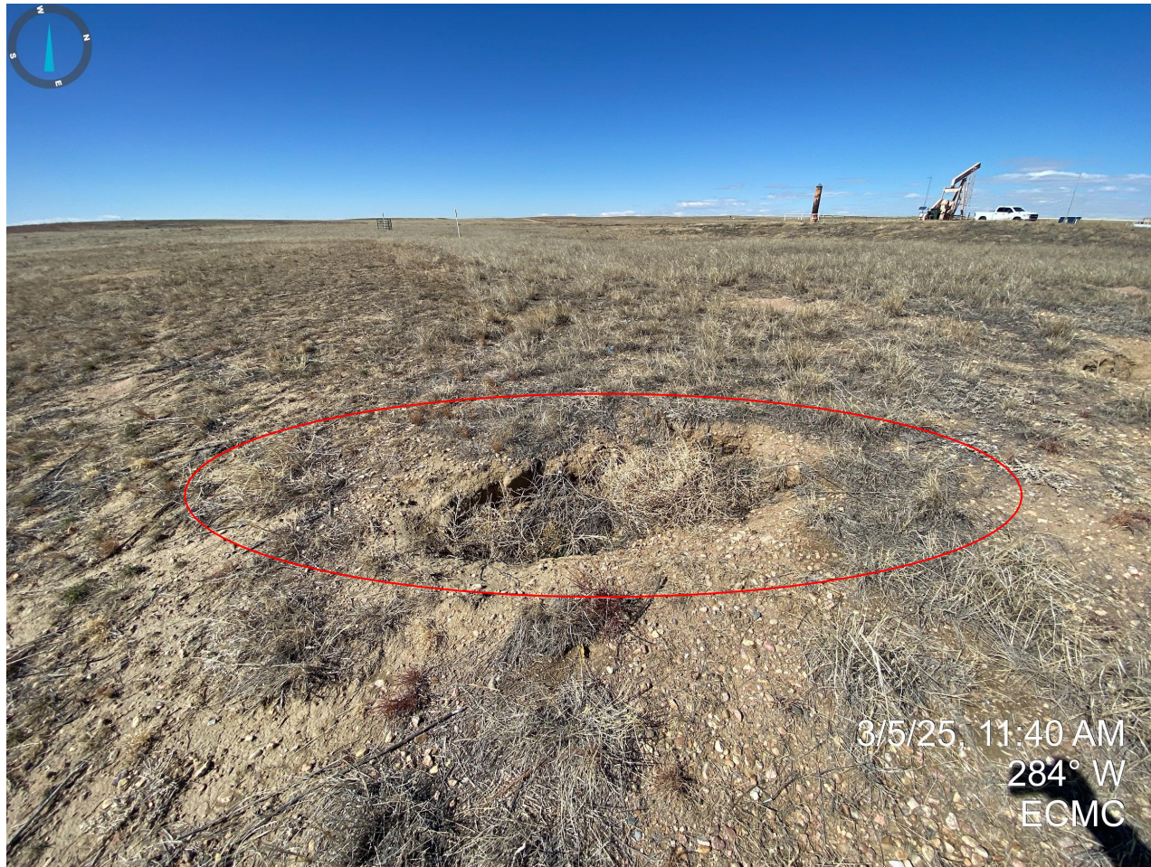
Photo 2. Subsidence observed on the west side of the former location entrance.
