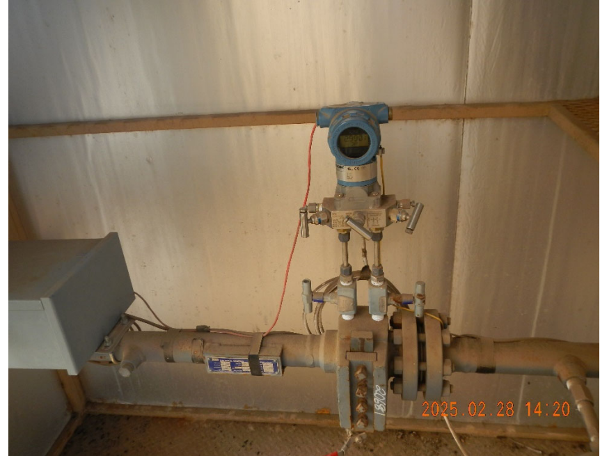
4. Gas meter inside meter shed.
