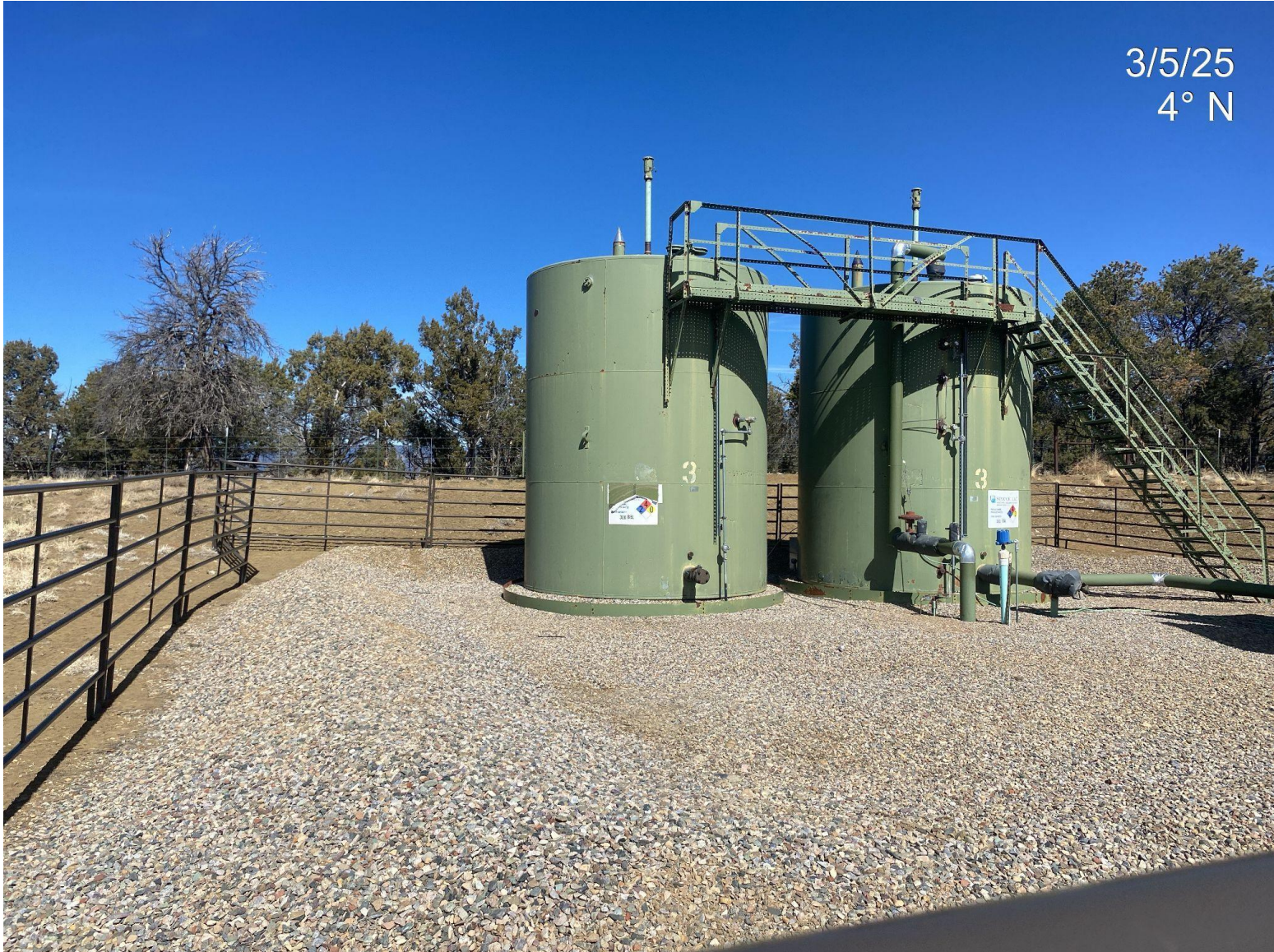
Photo 3. Produced water tank label is peeling and illegible.
