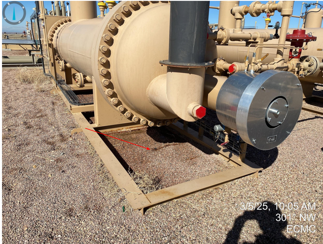
Photo 2. Stained soil observed under separator.
