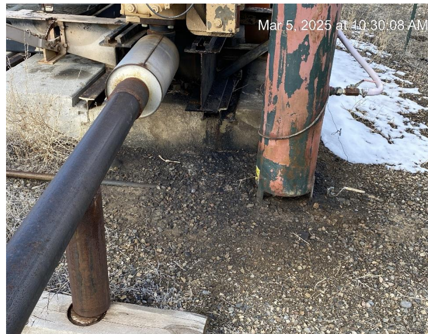
Lube oil staining
