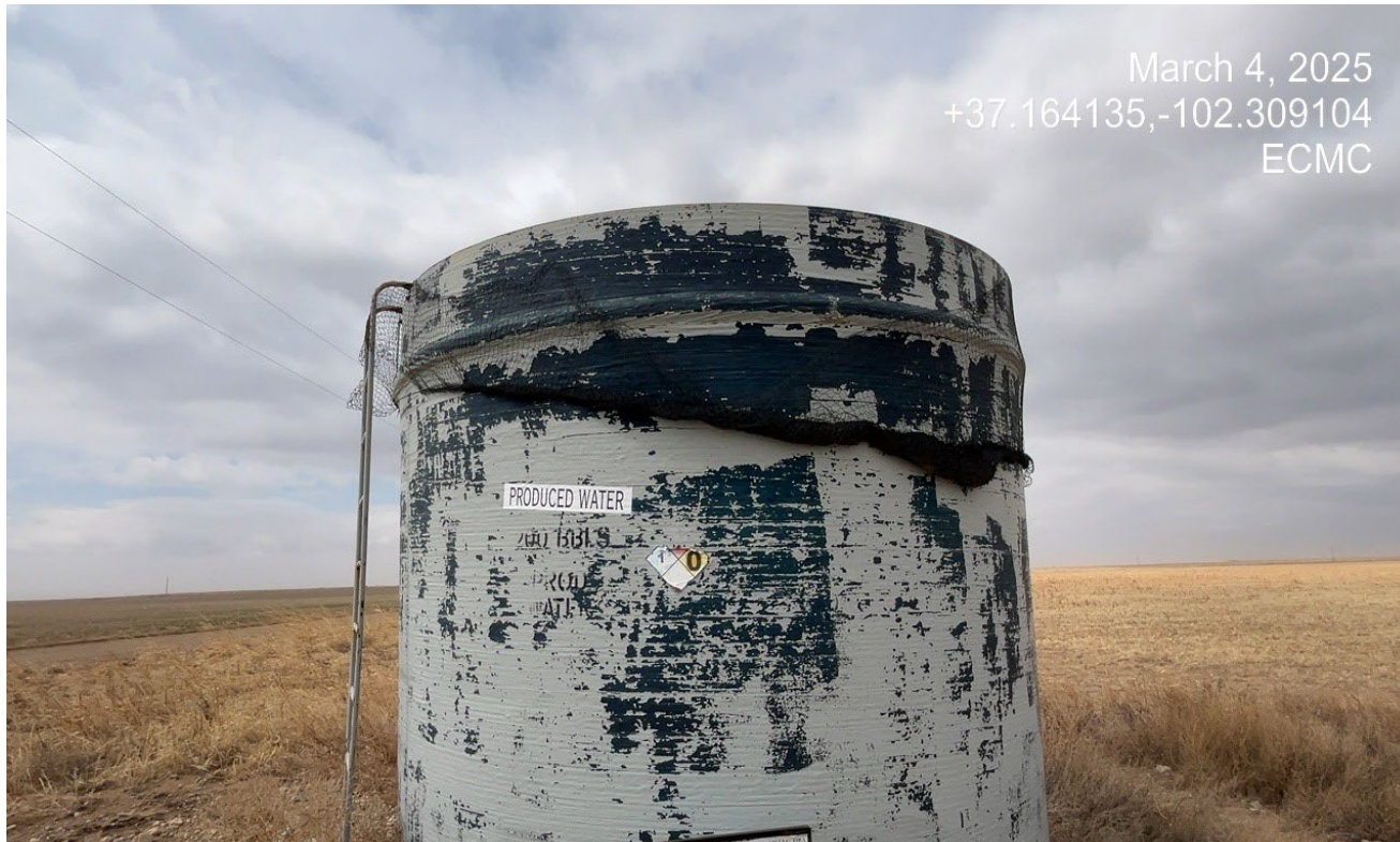
Photo 2. The netting on the tank is not maintained to prevent wildlife entry.
