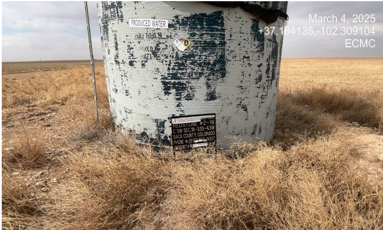
Photo 3. The secondary containment is insufficient to contain a spill and there are weeds around the tank.
