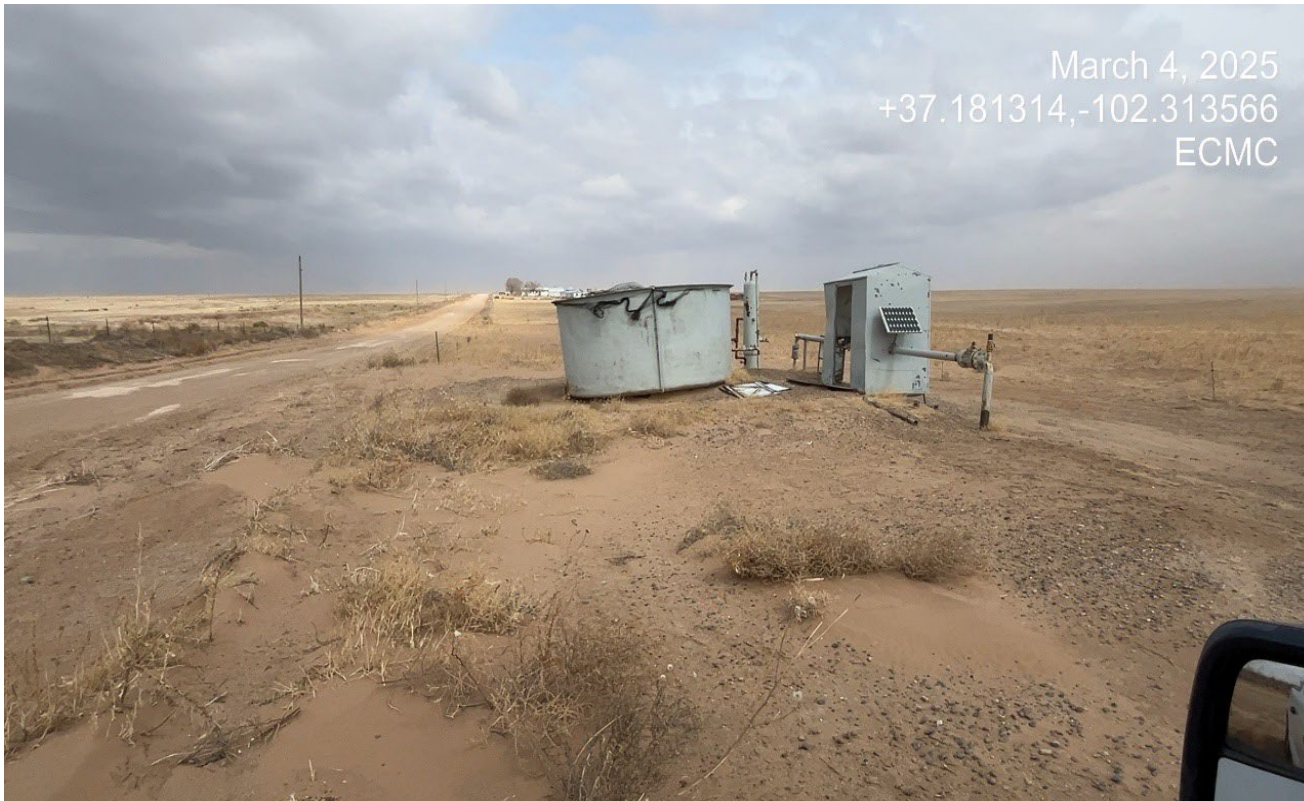
Photo 1. Facing north toward the offsite tank battery. The tank does not have sufficient secondary containment.
