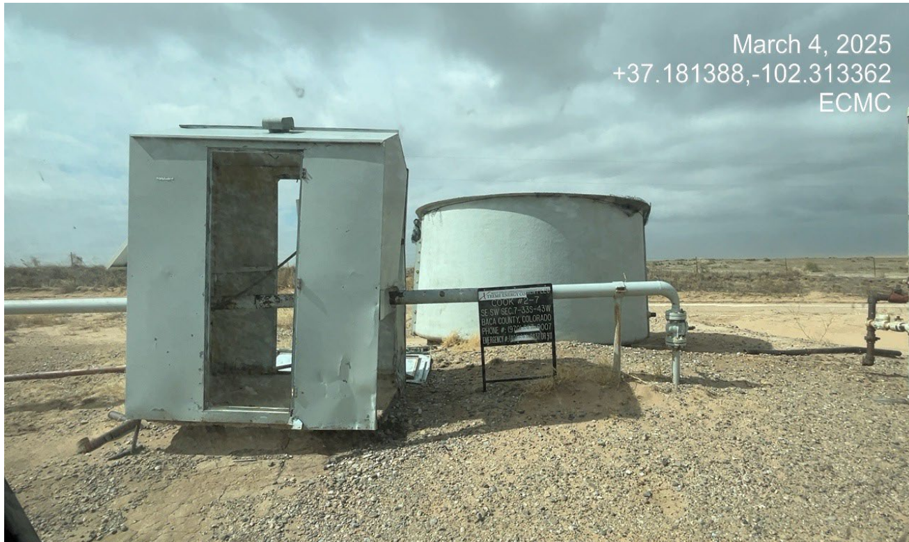
Photo 2. The sign is posted at the back side of the tank. The meter shed door has fallen off.
