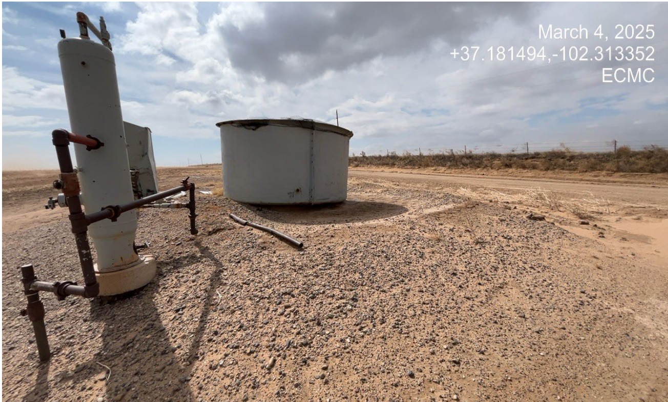
Photo 3. The tank does not have sufficient secondary containment.
