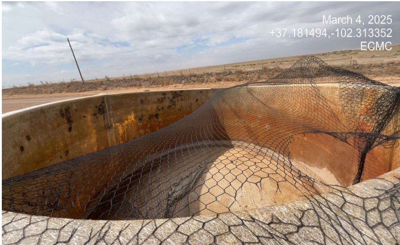
Photo 4. The netting on the tank is not maintained to prevent wildlife entry.
