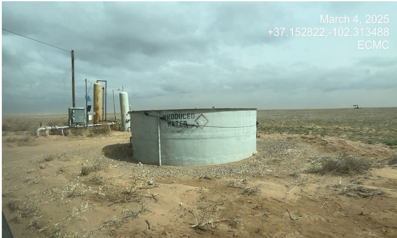
Photo 1. Facing northeast toward the offsite tank battery. The tank does not have sufficient secondary containment and the labels are missing.
