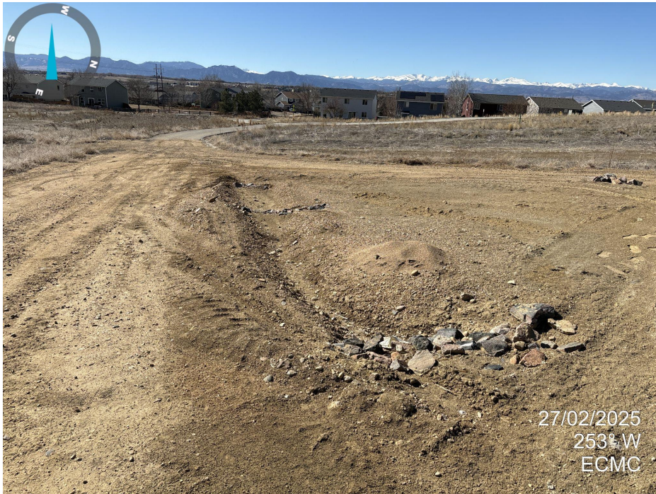
Photo 9. Looking west across the former tank battery in the center part of location. Check dams are present, dams are full of sediment.
