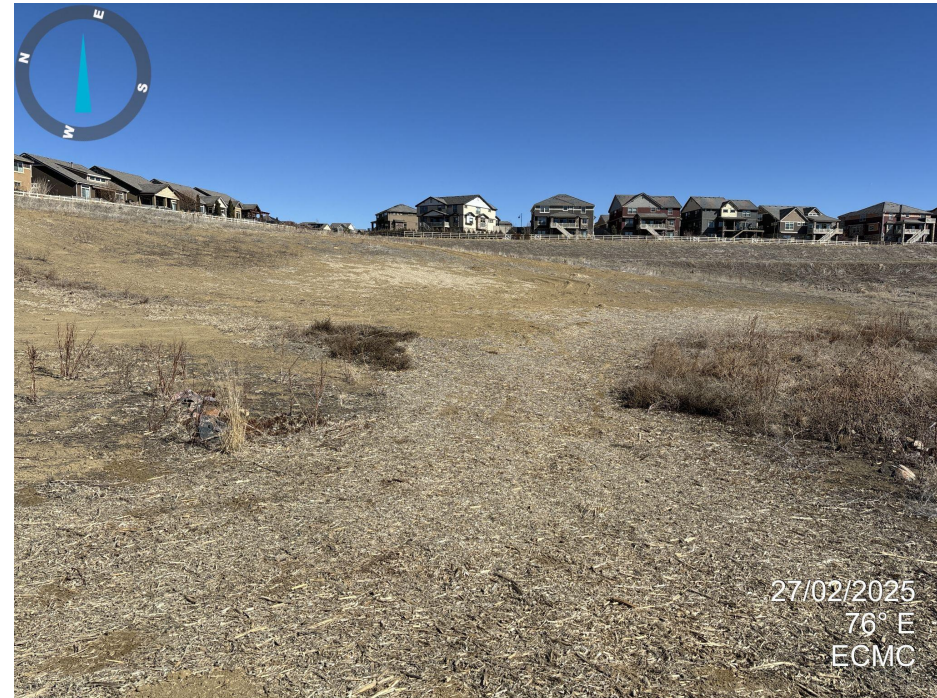
Photo 6. Looking east from the edge of the pad. Stormwater BMPs (rock check dams) are present in this area. Corn/straw cover is present in this area. At the time of inspection no germination was observed and ground was primarily bare soil. Undesirable weeds Kochia and Russian thistle are present in the areas around the well pad.
