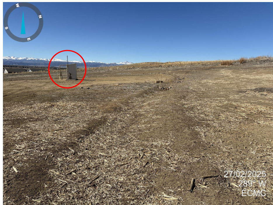
Photo 8. Looking west across the north side of pad. A perimeter ditch with rock check dams is in place. Shed with pipe riser remains on location (red circle), also pictured in Photo 4.
