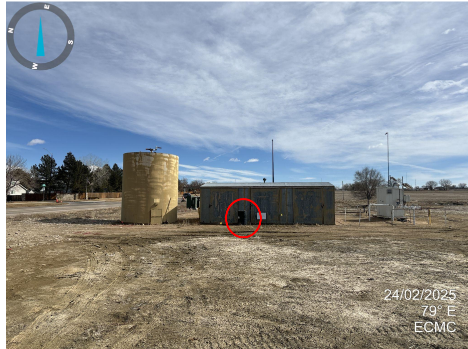
Photo 6. Looking at the east side of location. Chemical barrel outside of secondary containment (red circle).
