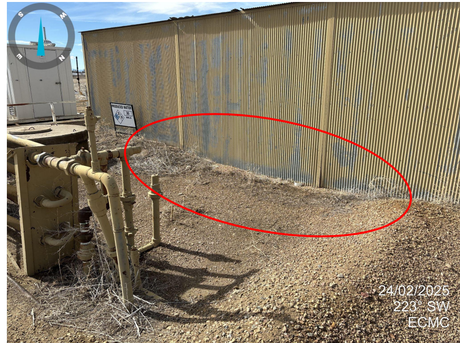
Photo 10. Secondary containment around partially buried produced water vessel is insufficient. The western side does not have a gravel berm and liquid could run out through the gap in the shed wall (red circle).
