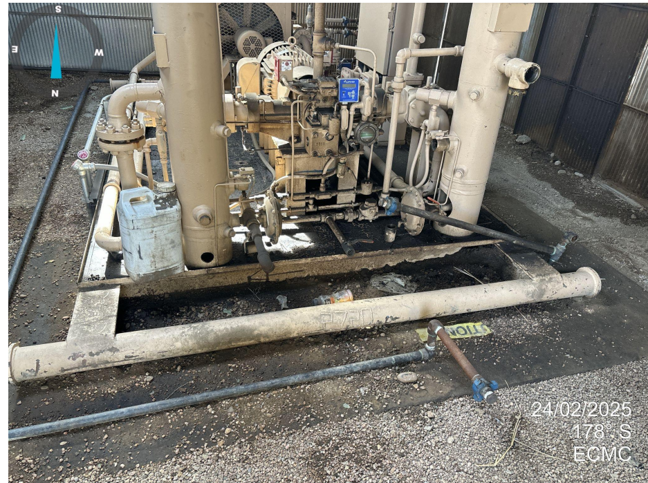
Photo 8. Inside shed, oily waste is present around equipment.
