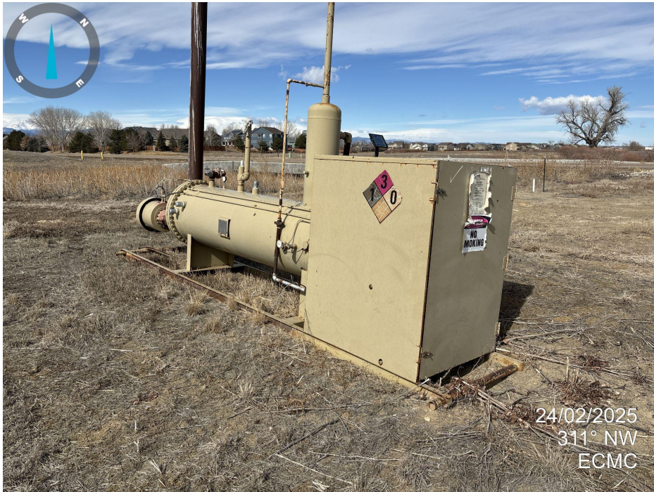
Photo 3. Separator on west side of location. Appears to be unused.
