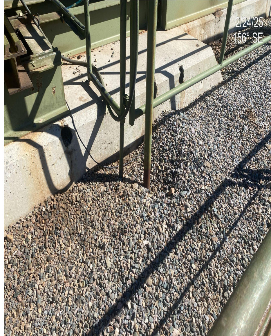
Photo 2. Spill prevention installed at oil tank is not sufficient.
