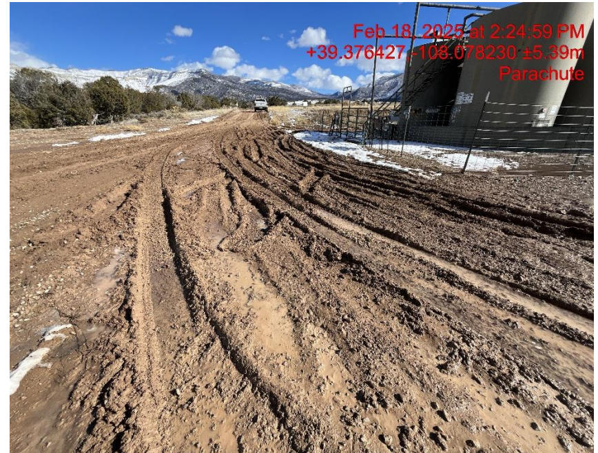
Photo # 5310 Lack of stabilization/compaction on location and lease road/insufficient tracking BMP's
