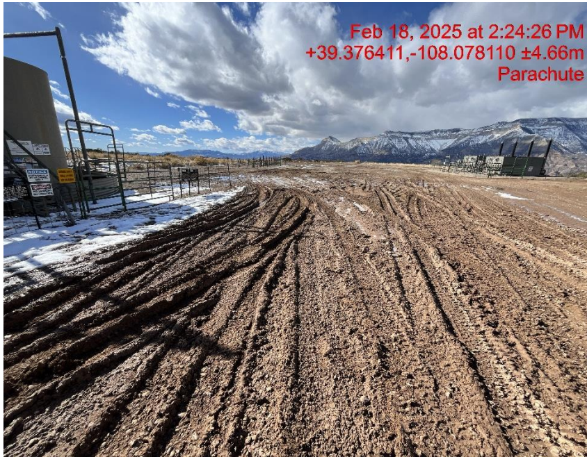
Photo # 5309 Lack of stabilization/compaction on location and lease road/insufficient tracking BMP's
