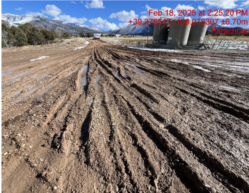
Photo # 5311 Lack of stabilization/compaction on location and lease road/insufficient tracking BMP's
