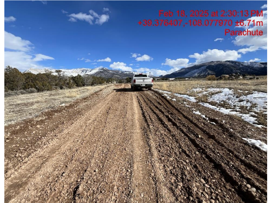
Photo # 5316 Lack of stabilization/compaction on location and lease road/tracking onto lease road/insufficient tracking BMP's
