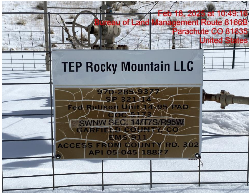
Weathered and Illegible Wellhead Sign – Photo #06673
