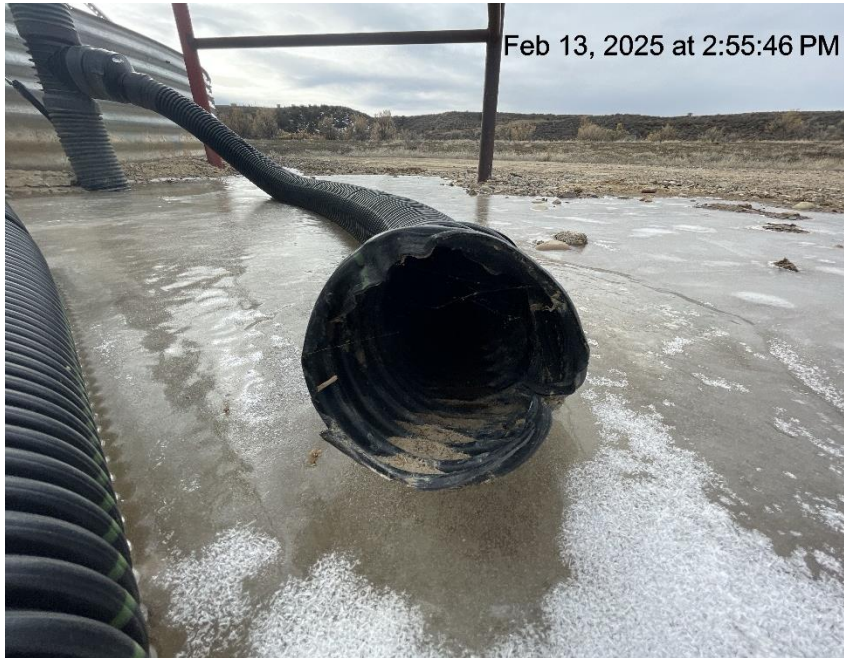
Photo # 6020 Flowline heating insulation open ended /wildlife hazard/available for entry by wildlife
