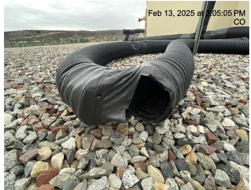
Photo # 6021 Flowline heating insulation damaged/wildlife hazard/available for entry by wildlife
