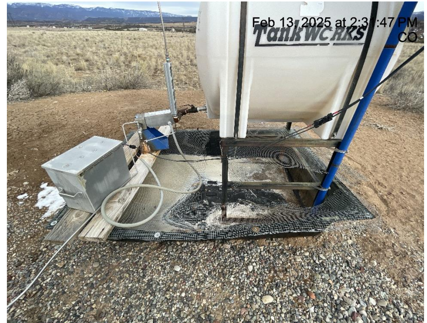
Photo # 5938 Wildlife protection on chemical tank containment needs maintenance/wildlife hazard
