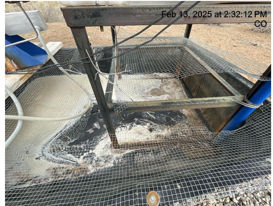
Photo # 5939 Wildlife protection on chemical tank containment needs maintenance/wildlife hazard
