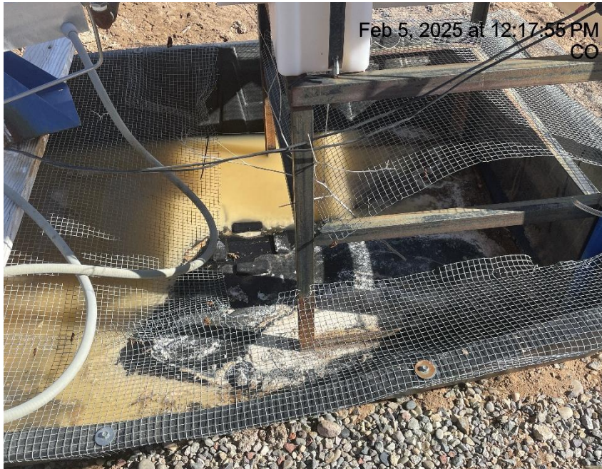
Photo # 3643 Wildlife protection on chemical tank containment needs maintenance/wildlife hazard
