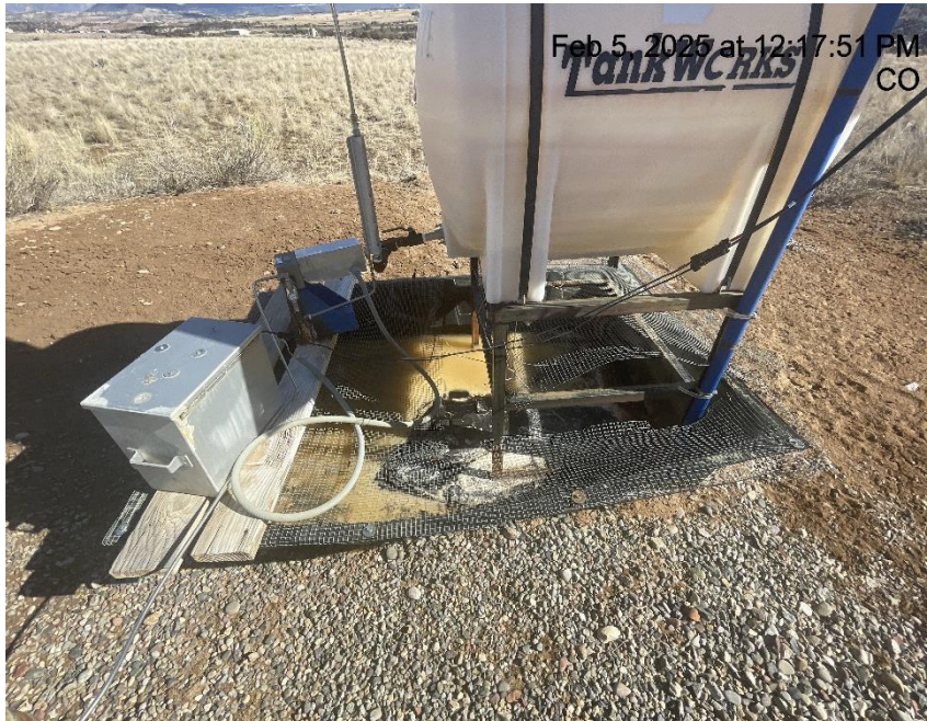
Photo # 3642 Wildlife protection on chemical tank containment needs maintenance/wildlife hazard
