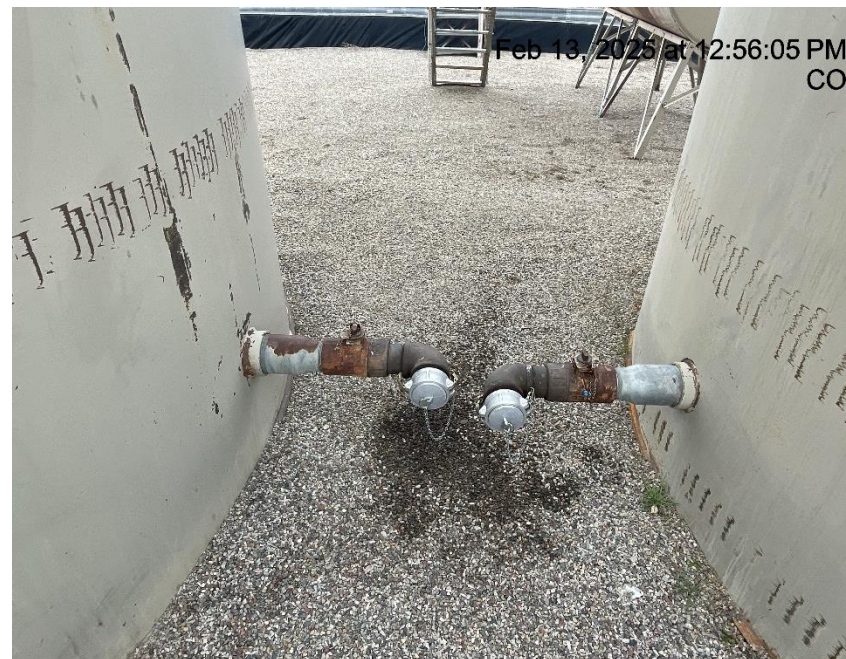
Photo # 5637 Small amount of staining in secondary containment
