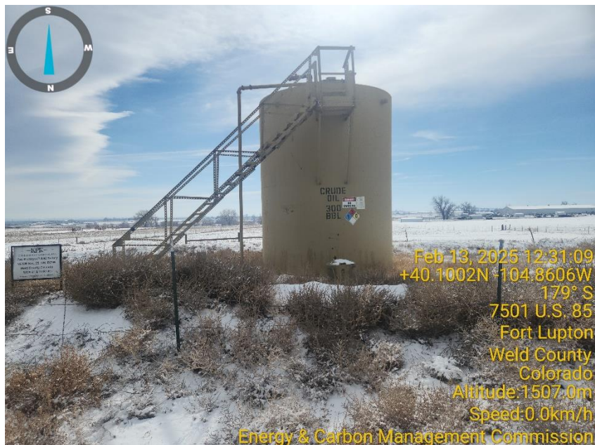
Photo 7 Tank battery, dead vegetation inside/outside tank battery fencing.
