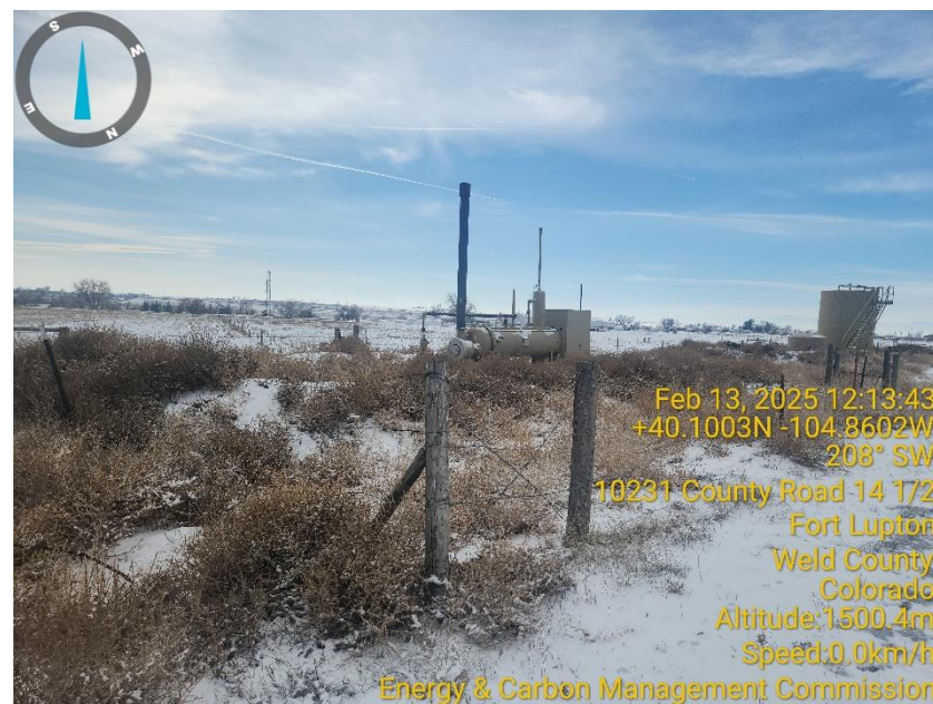
Photo 2 Dead vegetation around Horizontal Heated separator.
