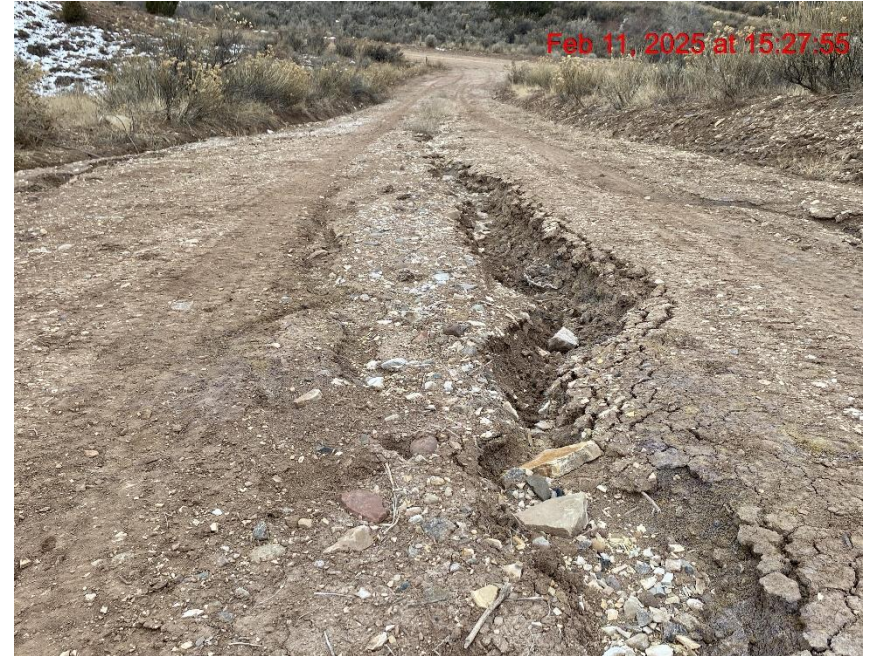
Rill Erosion on Access Road – Photo #06615
