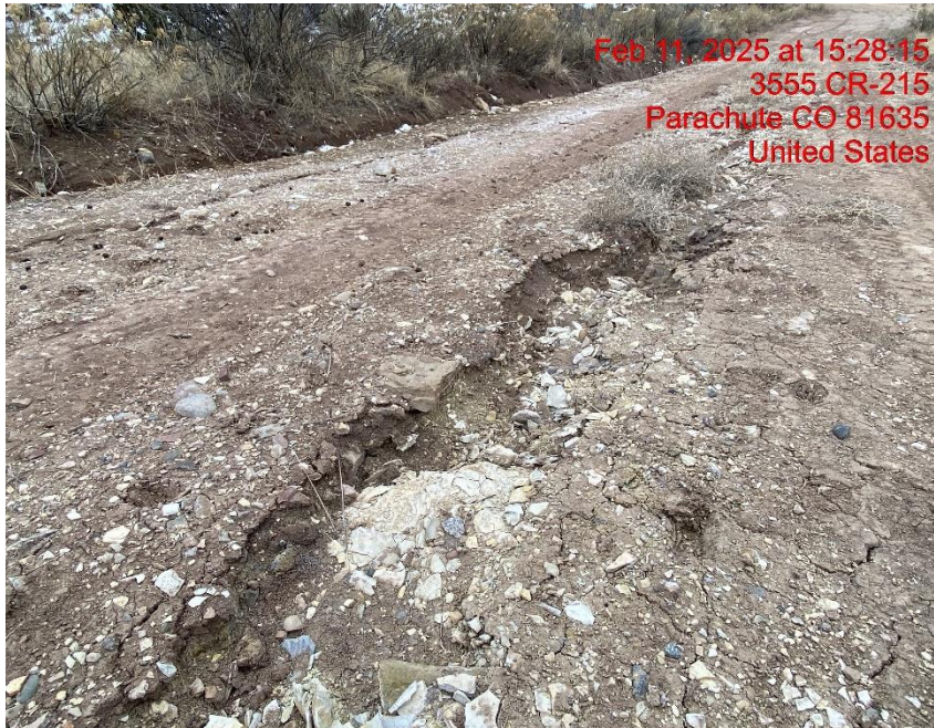
Rill Erosion on Access Road – Photo #06616
