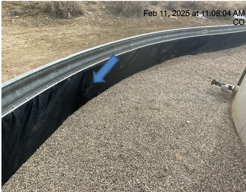
Photo # 5019 Hole in liner/liner needs maintenance
