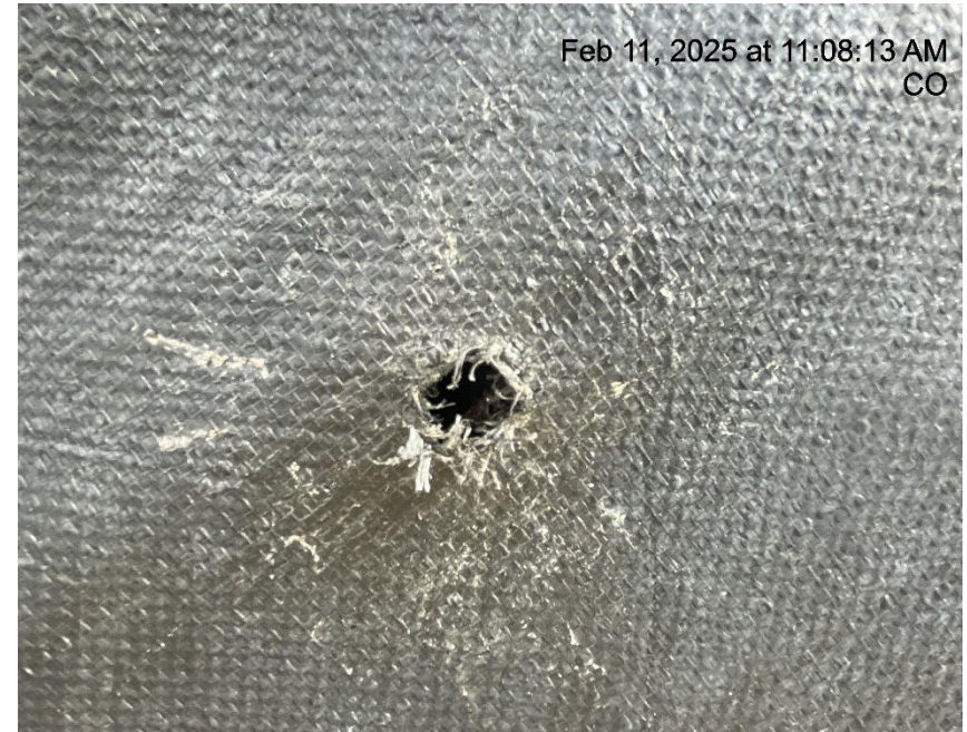
Photo # 5018 Hole in liner/liner needs maintenance
