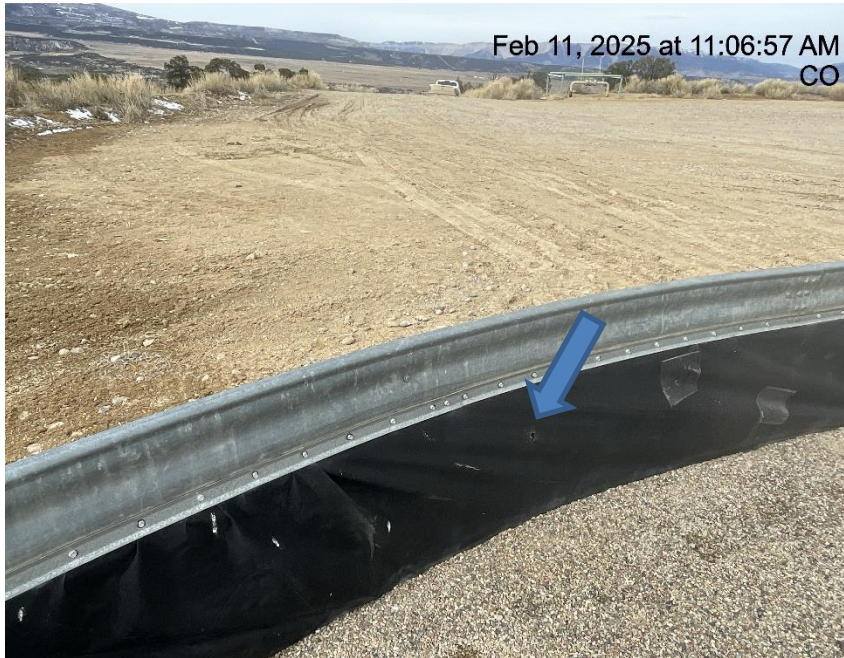
Photo # 5015 Hole in liner/liner needs maintenance
