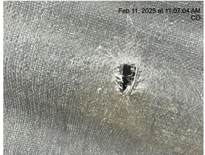
Photo # 5016 Hole in liner/liner needs maintenance
