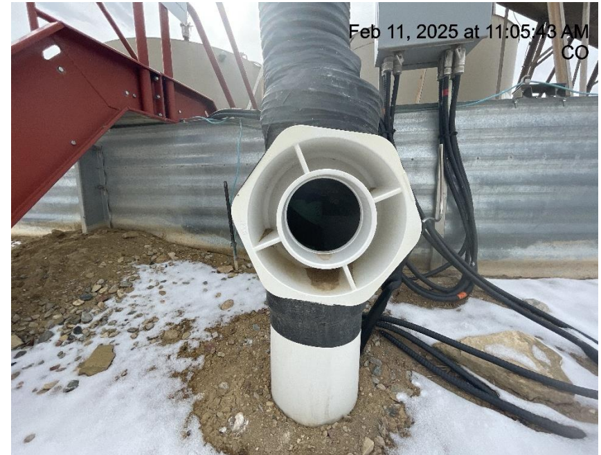
Photo # 5008 Flowline heating insulation open ended /wildlife hazard/available for entry by wildlife
