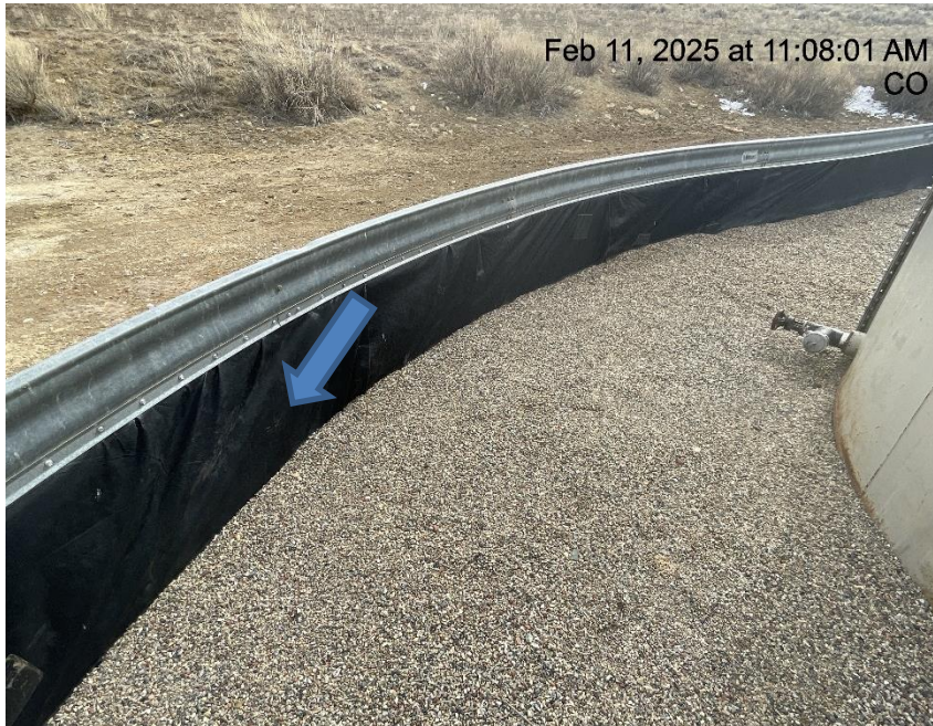
Photo # 5017 Hole in liner/liner needs maintenance
