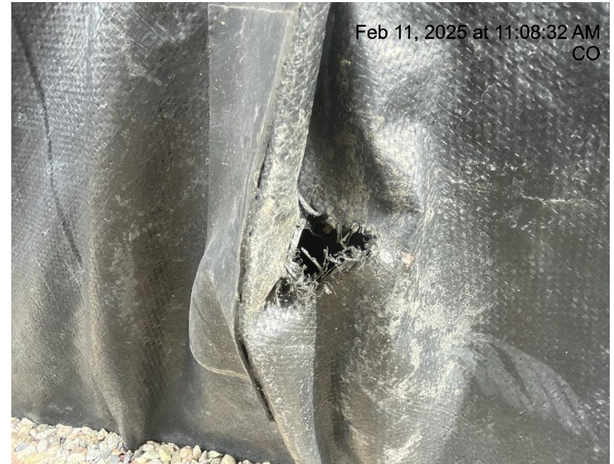
Photo # 5020 Hole in liner/liner needs maintenance
