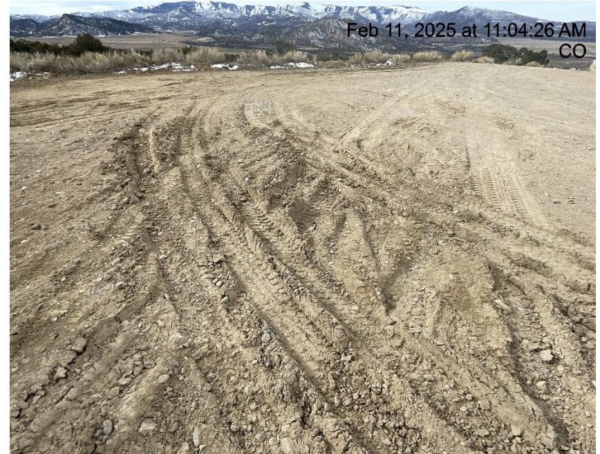
Photo # 5022 Lack of stabilization/compaction
