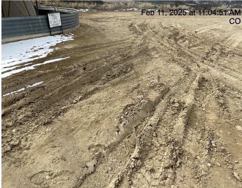
Photo # 5021 Lack of stabilization/compaction
