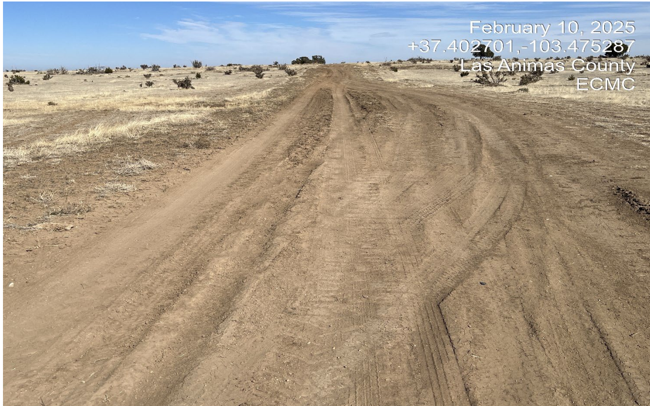
Photo 2. Facing northeast along the access road. There are areas of the road that will need to be repaired and stabilized. Vehicles are driving around the damaged area of the road.
