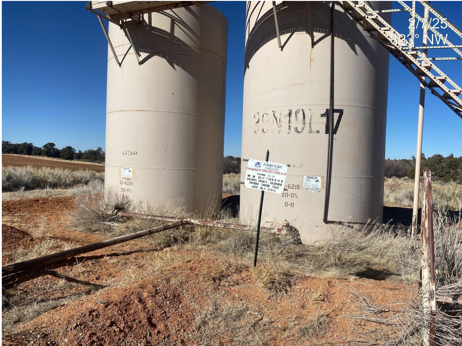
Photo 3. Weeds within tank berm. Note: new NFPA tank labels have been installed.
