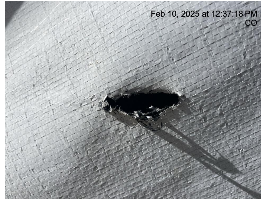
Photo # 4643 Hole in liner/liner needs maintenance
