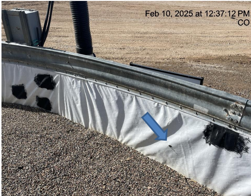
Photo # 4642 Hole in liner/liner needs maintenance
