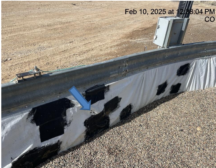
Photo # 4644 Hole in liner/liner needs maintenance
