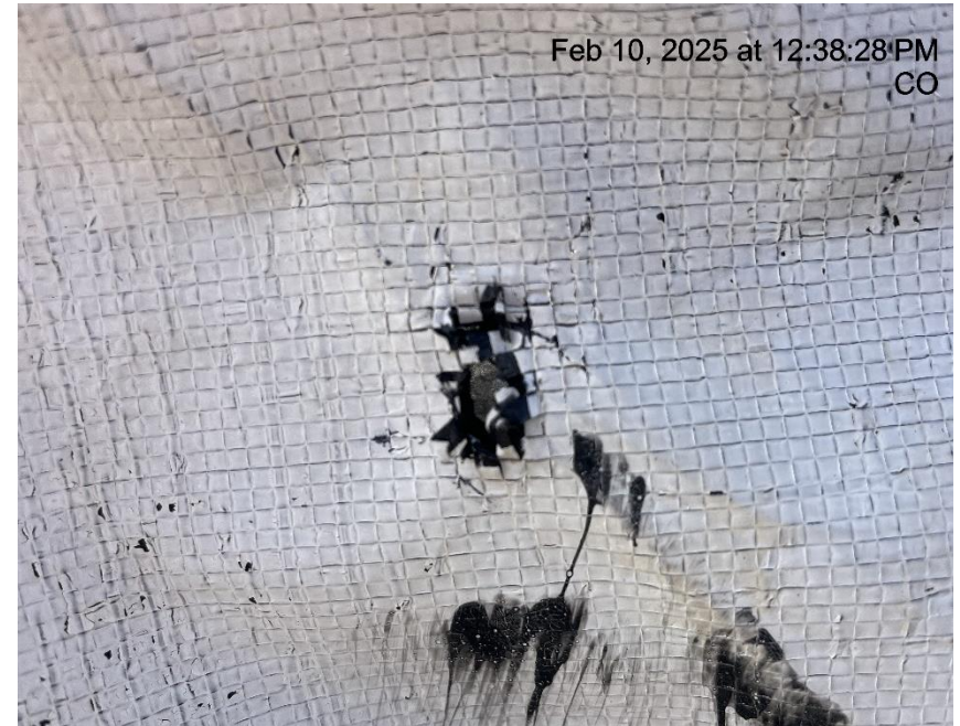
Photo # 4645 Hole in liner/liner needs maintenance
