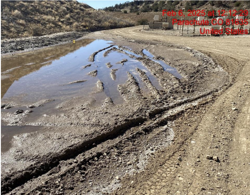
Lack of Stabilization – Photo #06523
