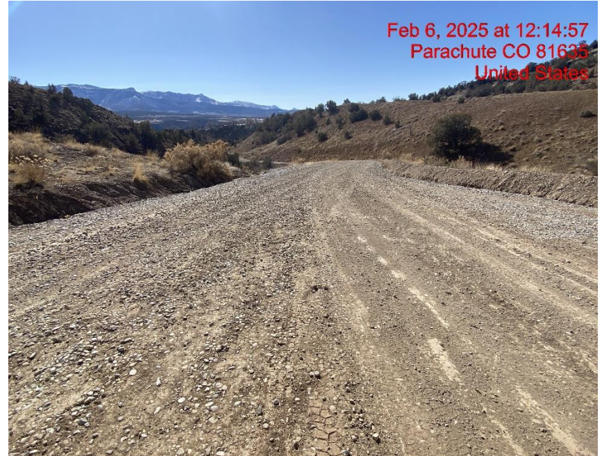
Insufficient Tracking BMPs – Photo #06524
