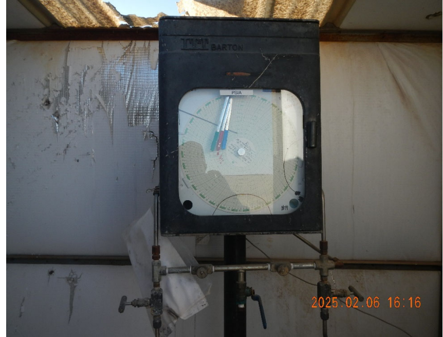
8. Gas meter inside meter shed.
