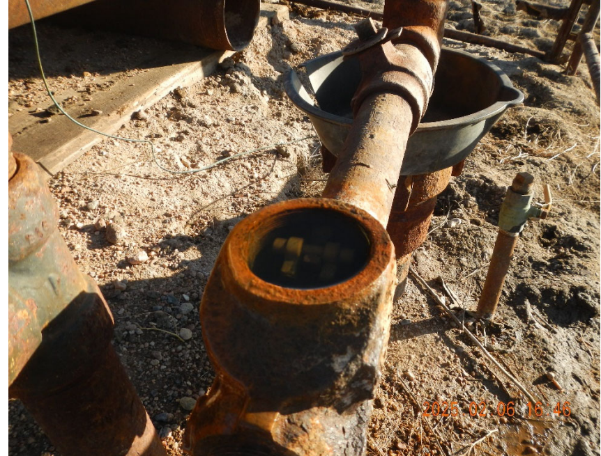
4. View of check valve with missing cap.
