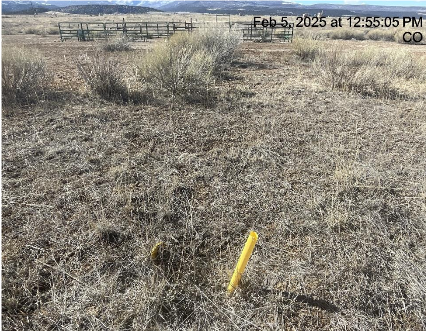
Photo # 3687 Improperly marked deadman
