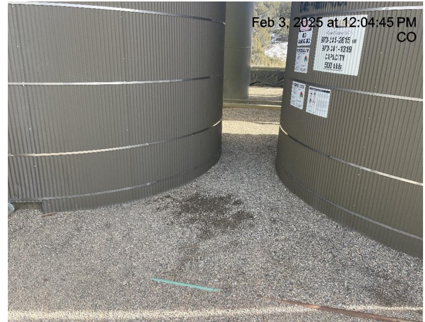
Photo # 3096 Staining in secondary containment
