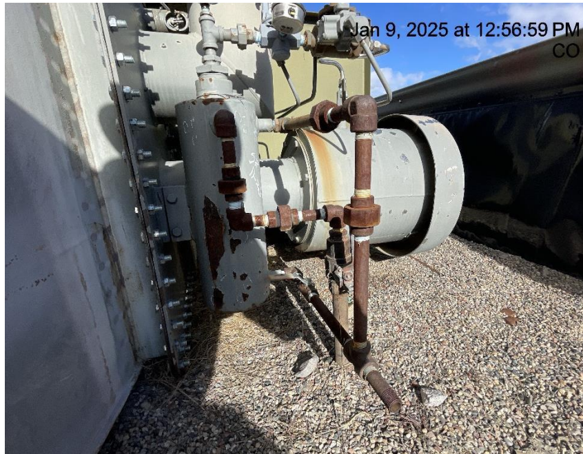
Photo # 7693 From inspection 708905468 conducted on 01/09/2025 PRV vent line does not comply with CECMC pressure safety device rules
