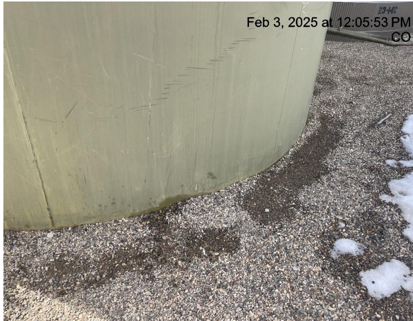
Photo # 3095 Staining in secondary containment
