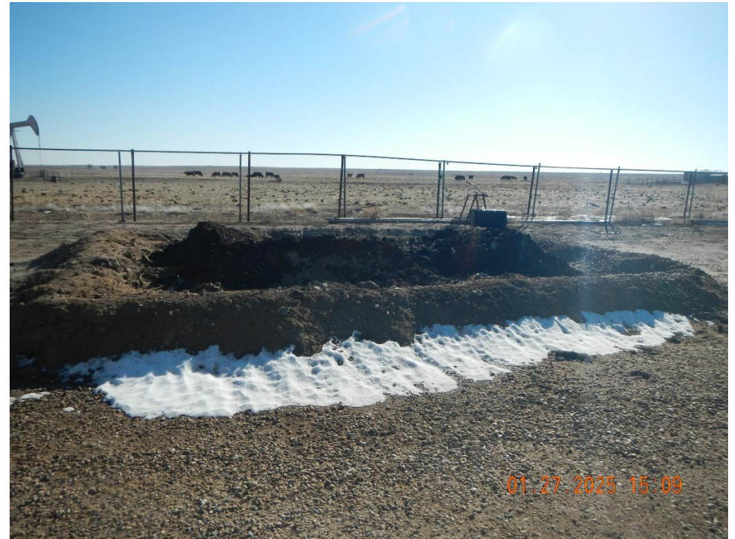
Contaminated material from spill being stored on location.
