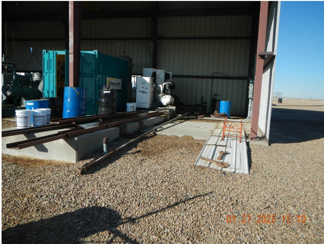
Stained ground around compressor equipment. Drums, buckets and jugs with no secondary containment.
