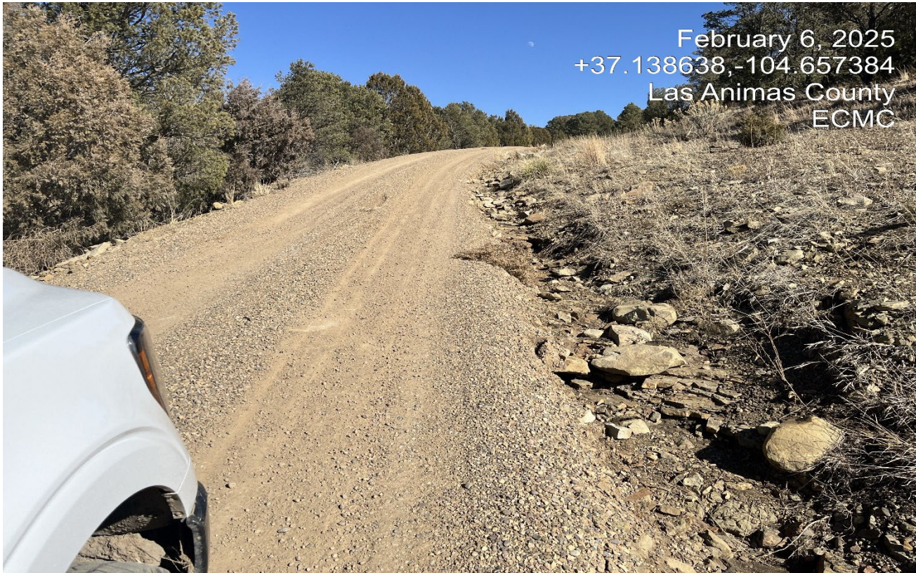
Photo 1. Facing northeast along the access road. There is a long stretch of road that concentrates stormwater down the roadside causing erosion.
