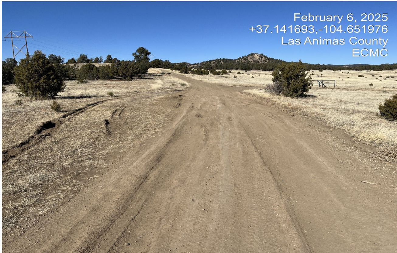
Photo 4. Facing north along the access road. This area of road is rutting and vehicle track went off road around this area. This area needs to be regraded.
