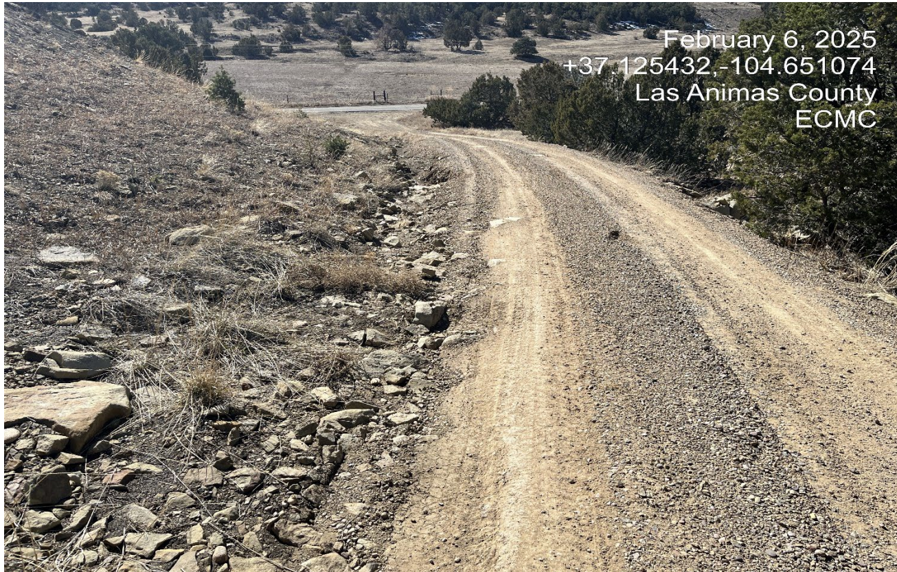
Photo 2. There is a long stretch of road that concentrates stormwater down the roadside causing erosion.
