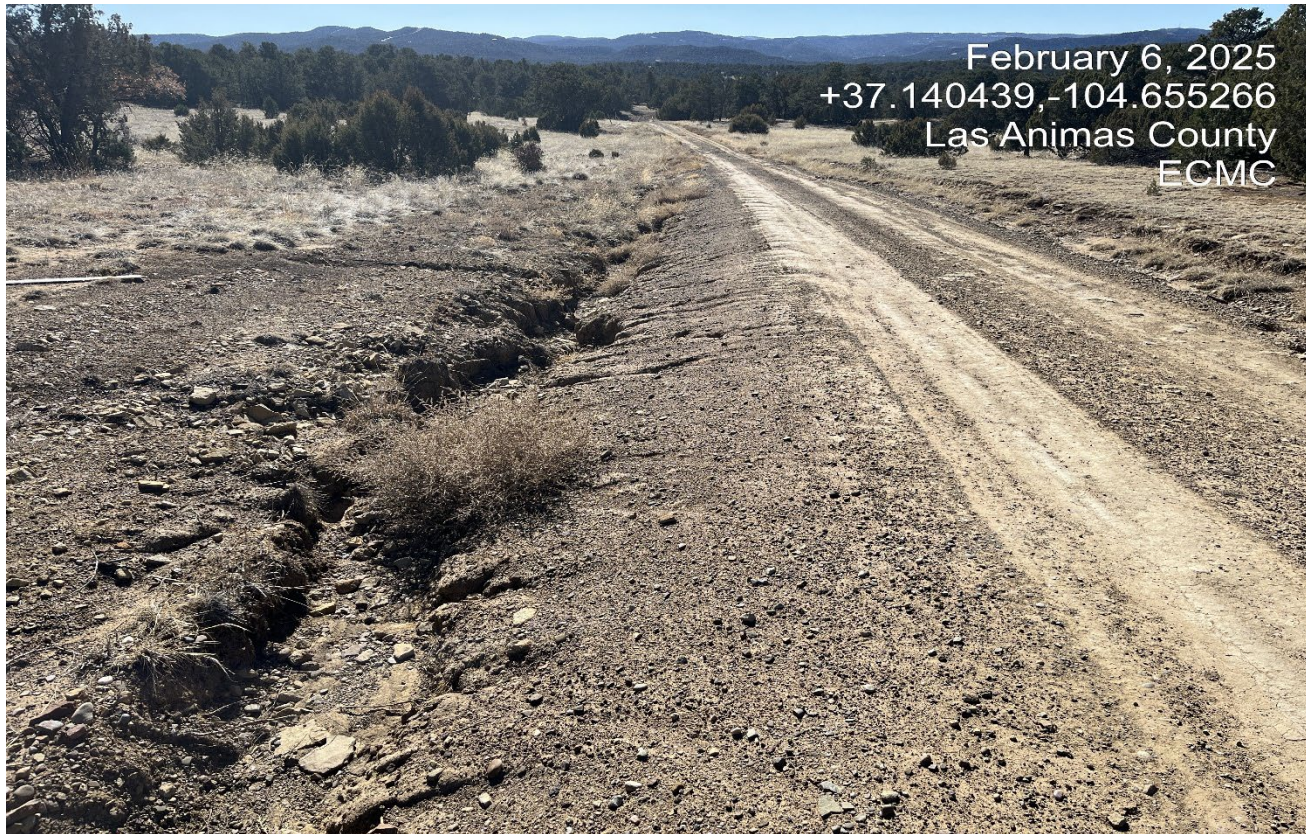
Photo 3. Facing southwest back down the access road. This area is eroded and needs to be repaired and stabilized.
