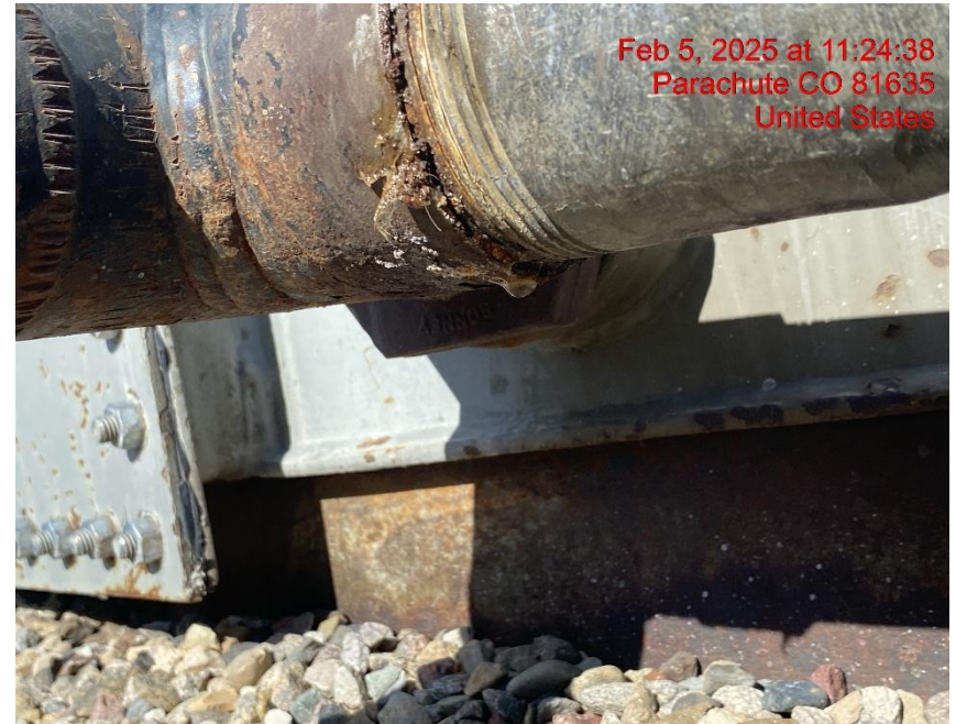
Leak at Valve Plug – Photo #06445
