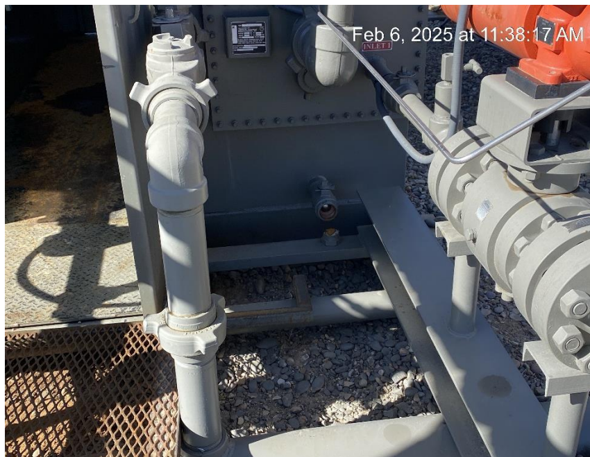
Open end ethylene glycol drain
