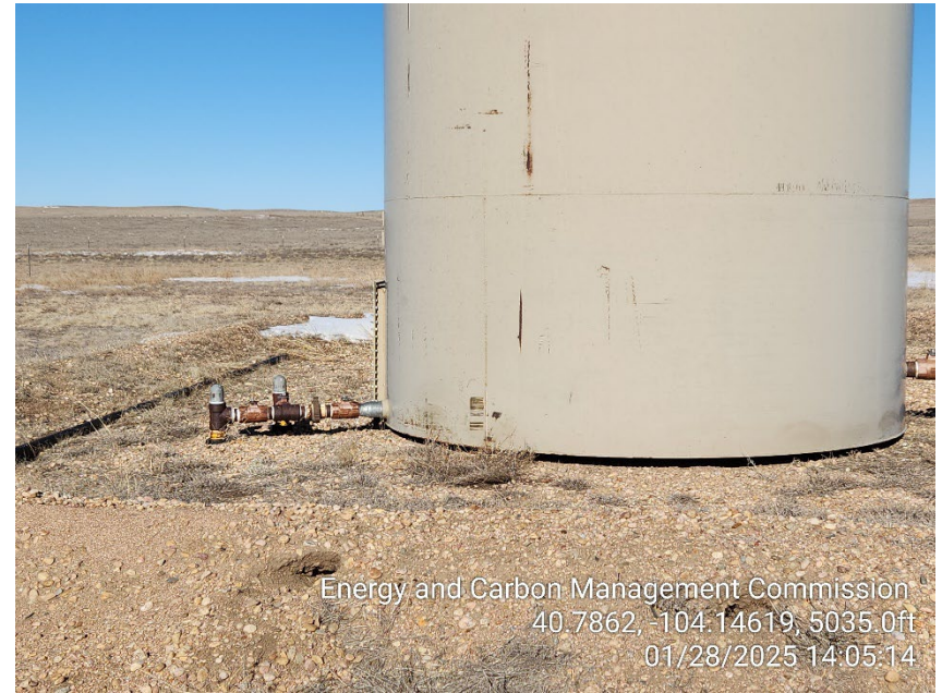
Photo 6 – Holes in Berm
