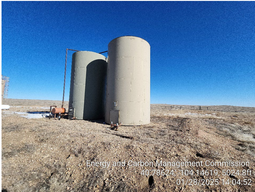
Photo 7 – Tank Battery
