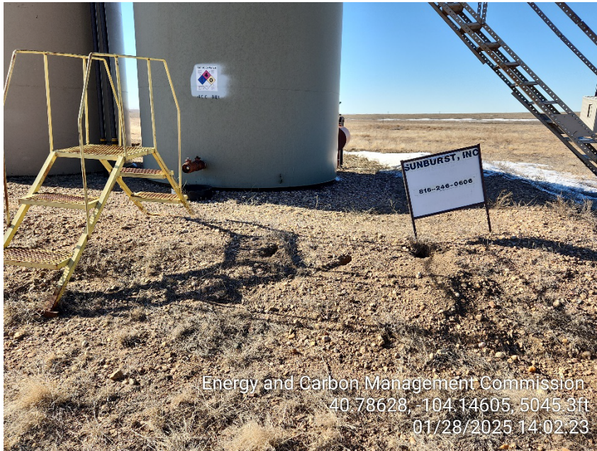
Photo 3 – Holes in Berm
