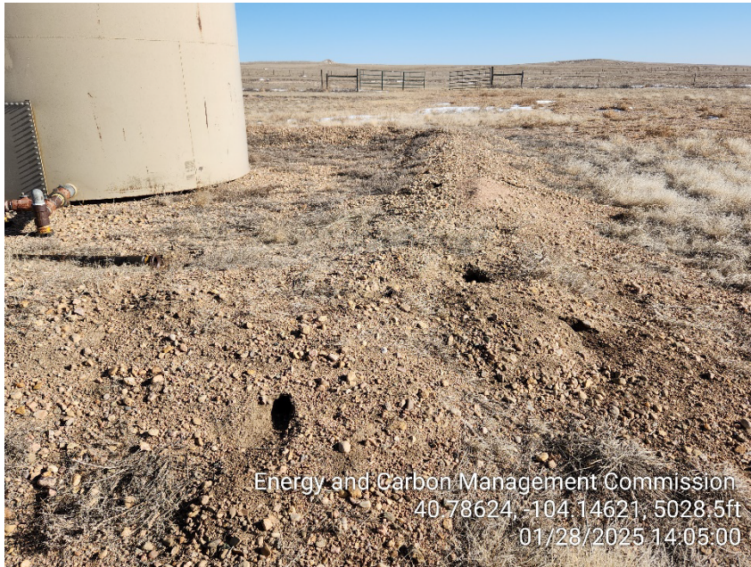
Photo 5 – Holes in Berm
