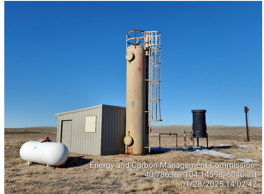
Photo 8 – Heater Treater, ECD, Flare and Propane Tank
