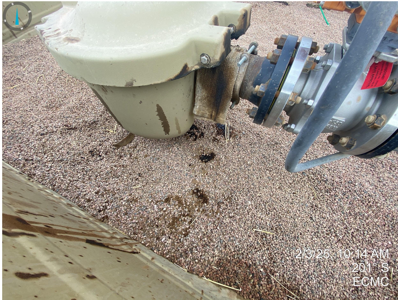
Photo 24. Continued from Photo 23; stained soil observed near loadout lines.
