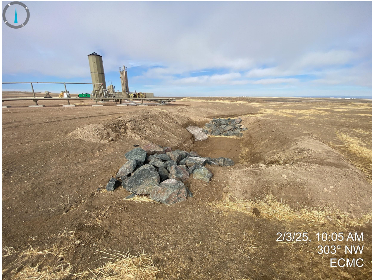
Photo 5. Sediment trap installed along the eastern side of the production facilities.
