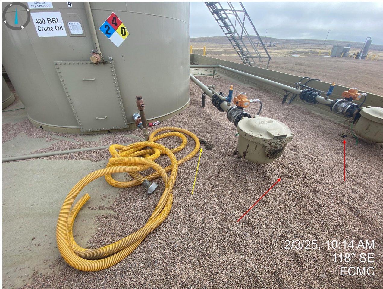
Photo 22. Stained soil observed near loadout lines, and oily rag (yellow arrow).
