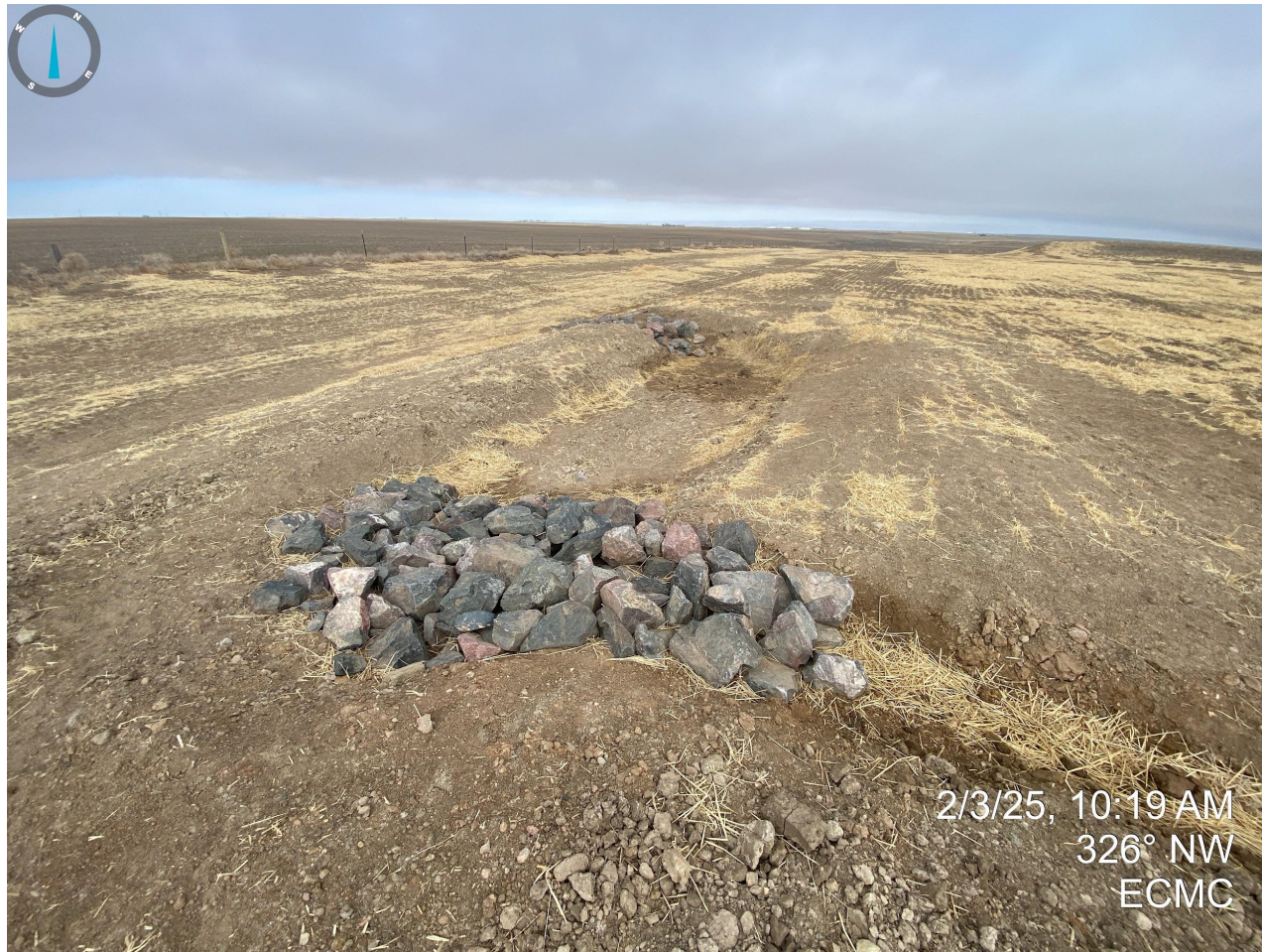
Photo 11. Sediment trap installed along the northwestern side of the production facilities.
