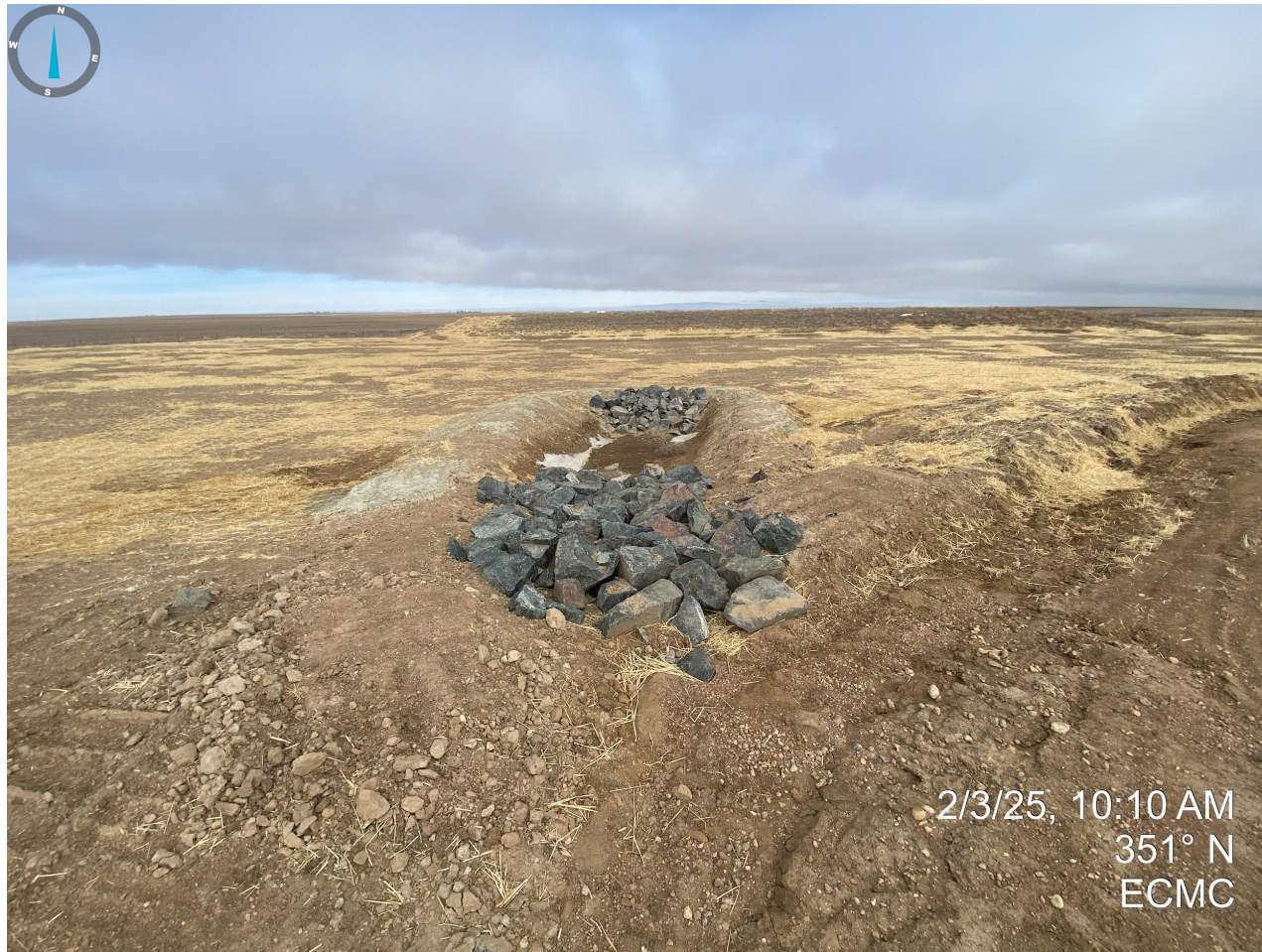
Photo 10. Sediment trap installed along the northern side of the production facilities.
