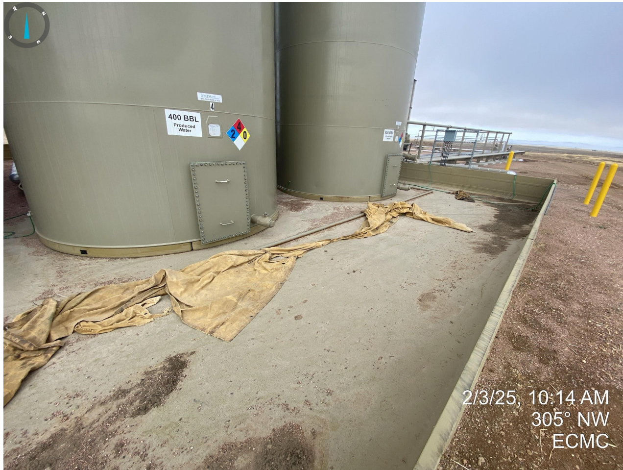
Photo 25. Trash/debris observed within tank battery secondary containment.
