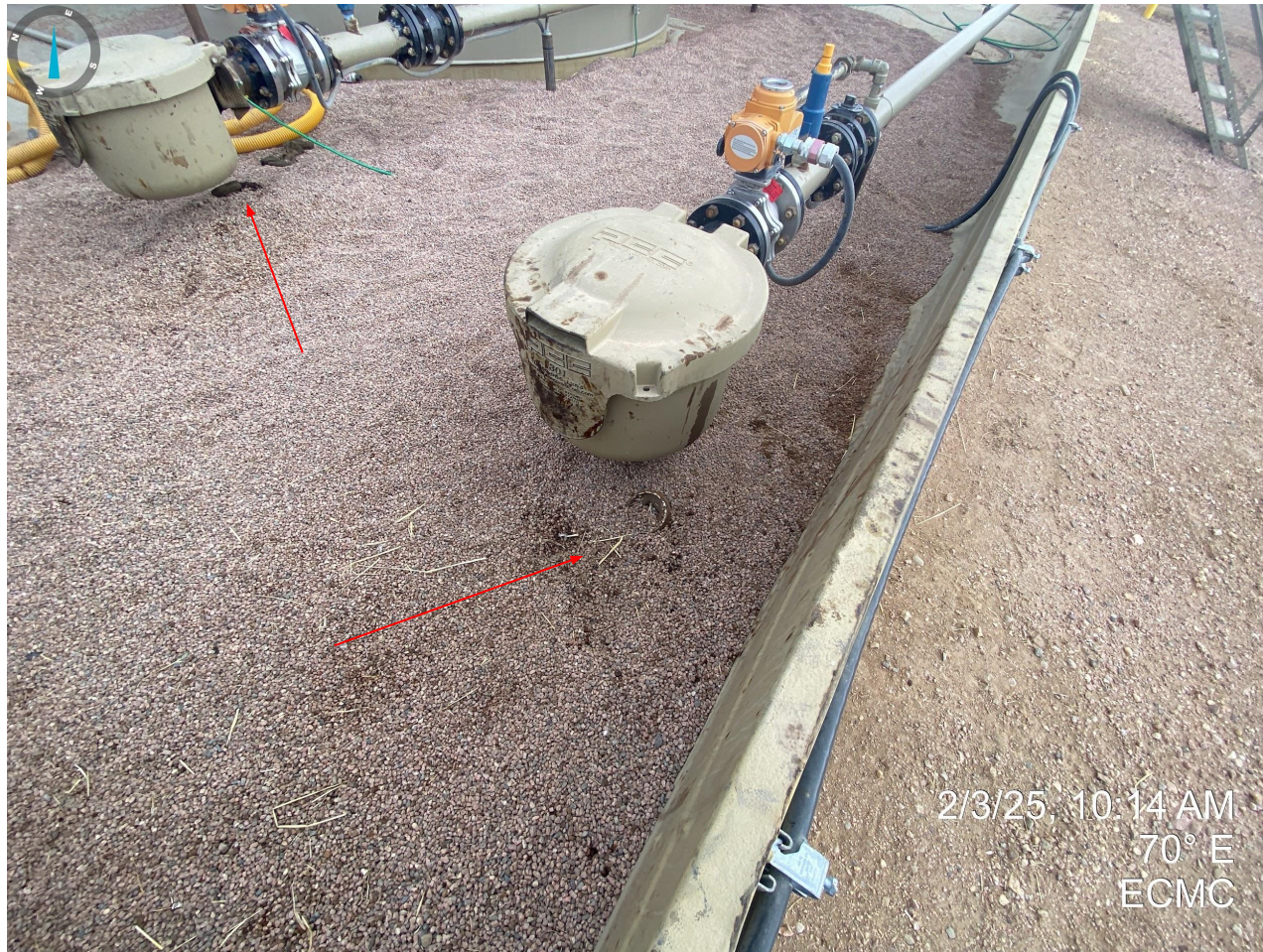
Photo 23. Continued from Photo 22; stained soil observed near loadout lines.
