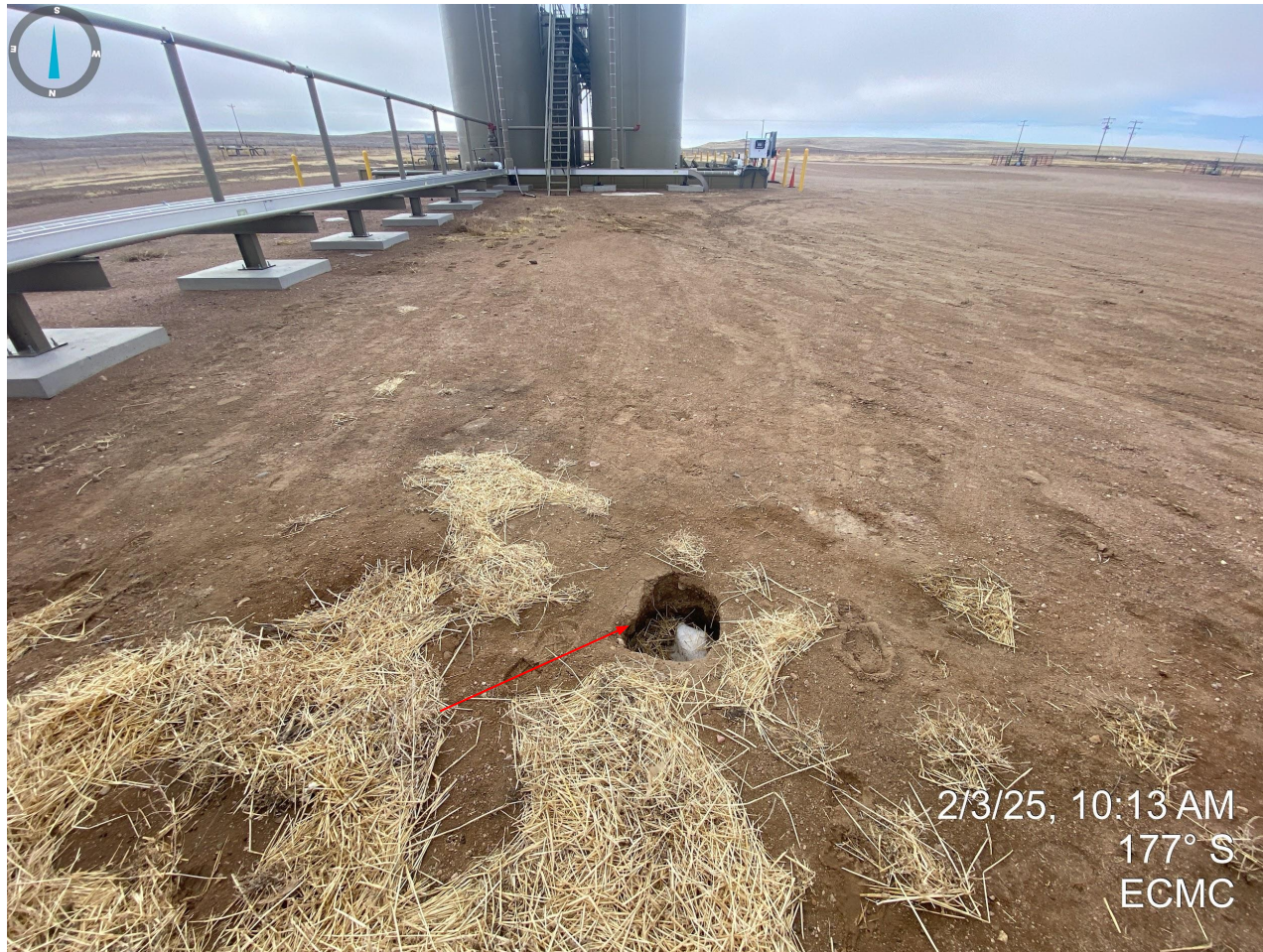
Photo 19. Pothole/subsidence north of tank battery.
