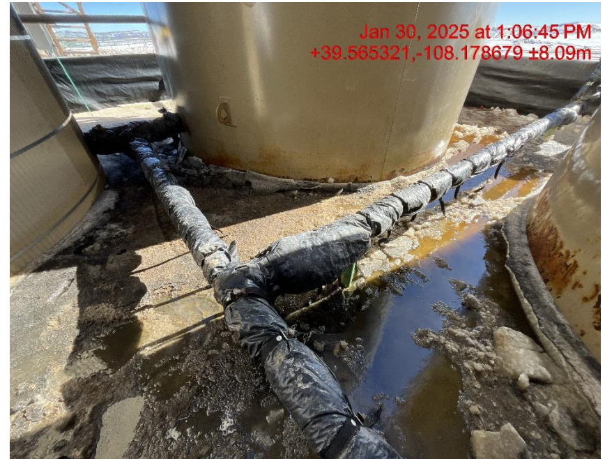
Photo # 3876 Staining in secondary containment
