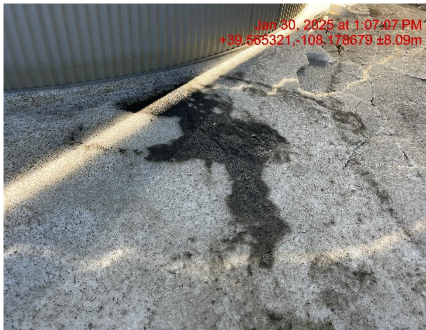
Photo # 3877 Staining in secondary containment
