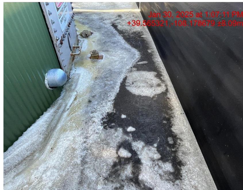
Photo # 3878 Staining in secondary containment
