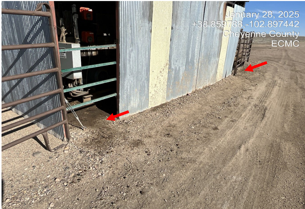
Photo 2. Facing toward the pumpjack engine shed. There are stained soils shown at red arrows that need to be cleaned up..
