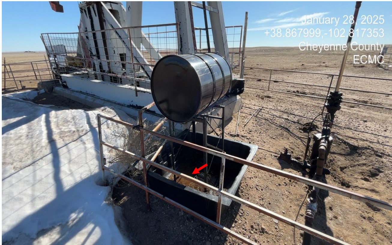
Photo 6. Facing toward the wellhead. The barrel has been repositioned into the secondary containment. There is oily fluids inside the containment and there are no wildlife protections to prevent entry.
