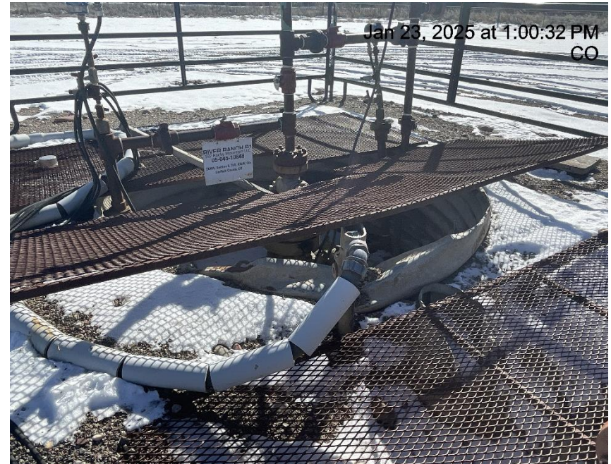
Photo # 1145 Cellar not properly covered/wildlife hazard
